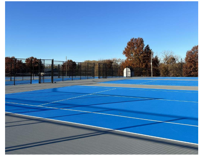
North Courts Looking Southwest
