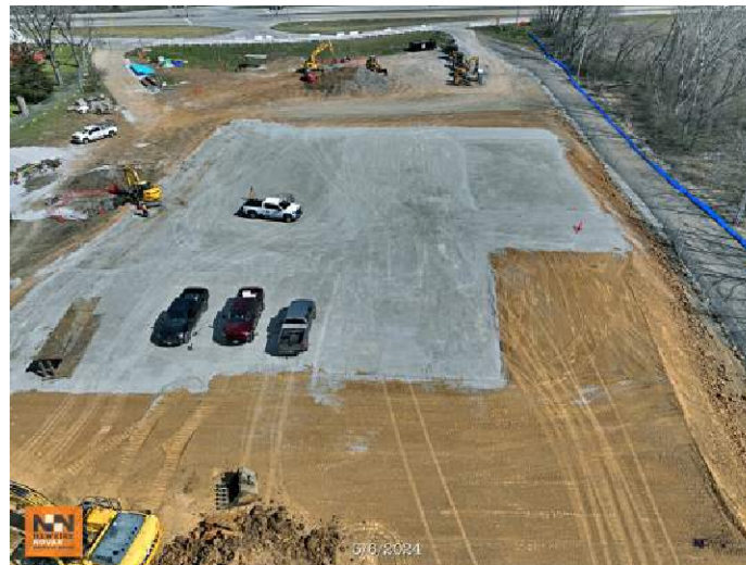
Overall Site/Building Pad
