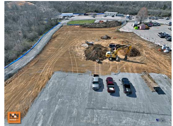
Overall Site/Building Pad
