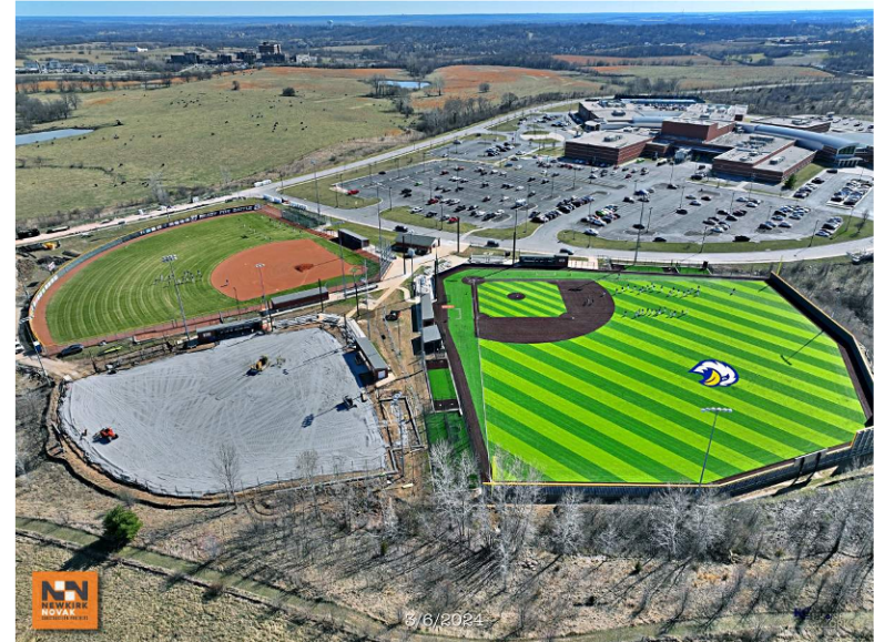
LNHS - Overall Site
