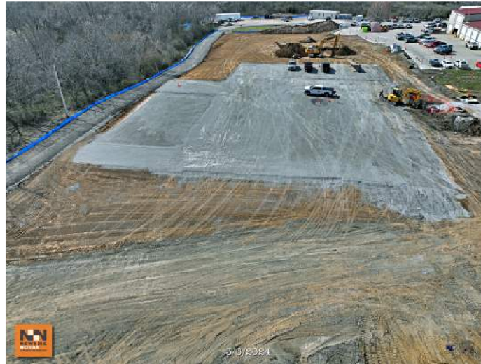
Overall Site/Building Pad
