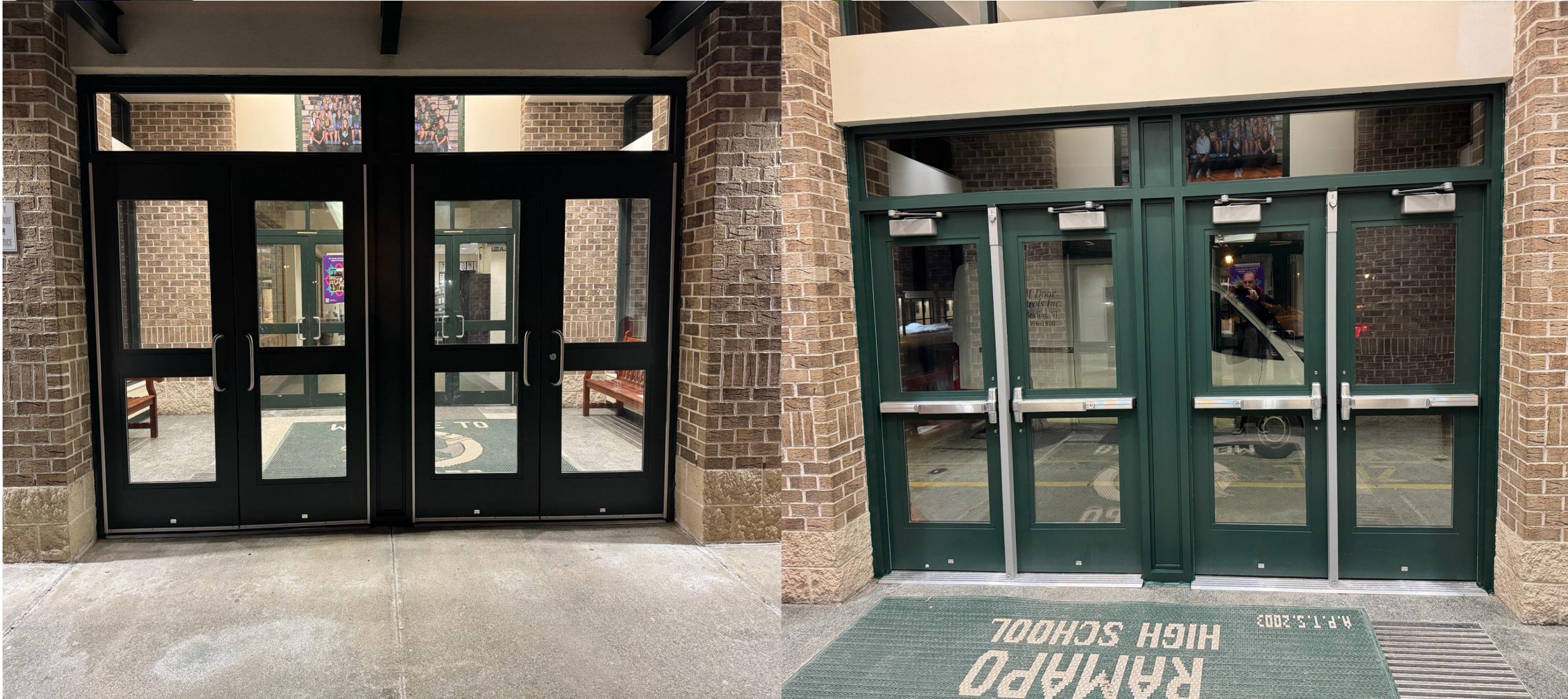
New Front Doors at RHS
