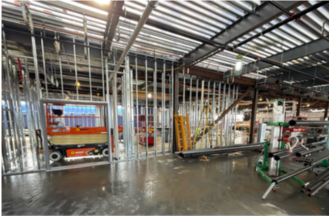
D Building Interior Framing
