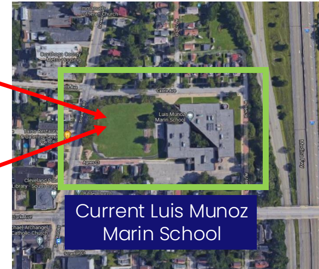
Former Lincoln High School - Location 3001 Scranton Rd (demolished 1977)
