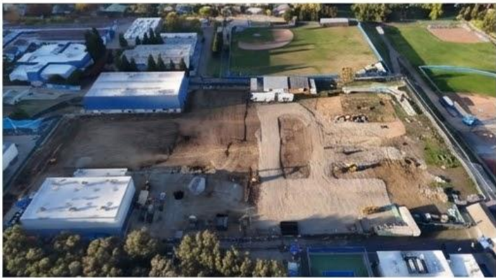
Foothill High School Building Pad for New Performing Arts Center
