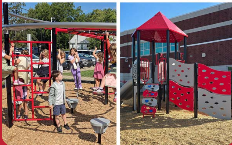
Construction on the new Gilles-Sweet Elementary playground kicked off as soon as the 2024-2025 school year wrapped up, and by Tuesday, Sept. 2, the wait was over. The first graders proudly took the first spin, climb, and swing on the brand-new equipment during its grand opening celebration.
