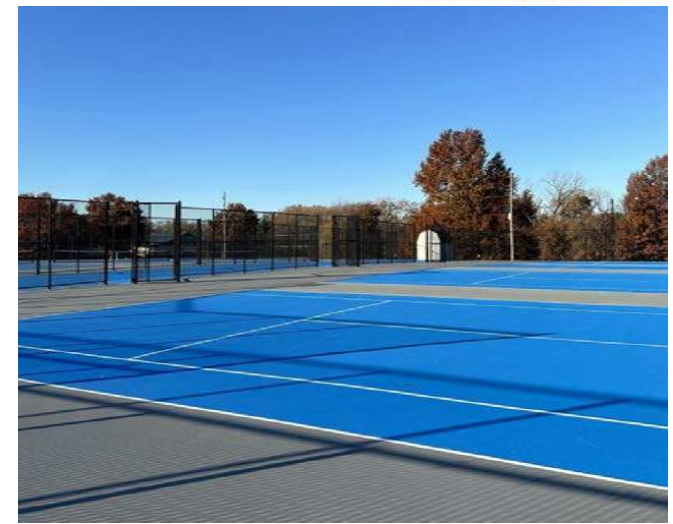
North Courts Looking Southwest
