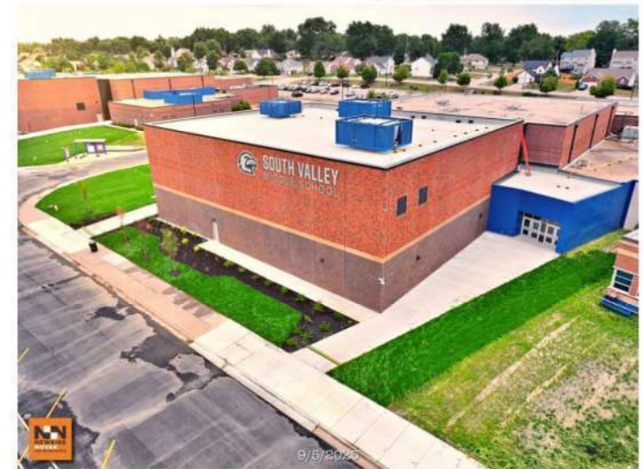
SVMS Exterior View
