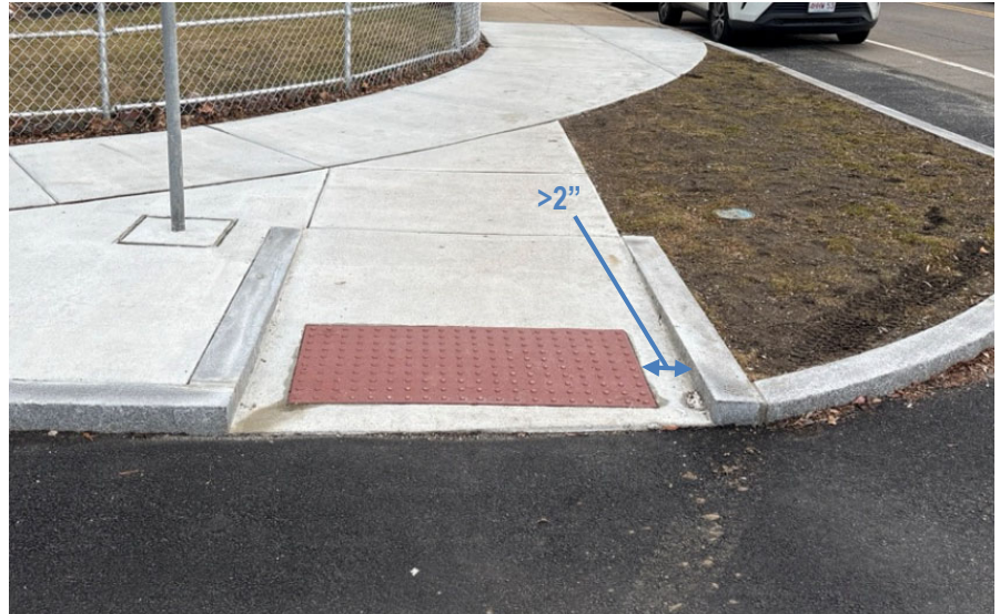
Ramp with insufficient DWP width at the intersection of Main St and Willard Ave
