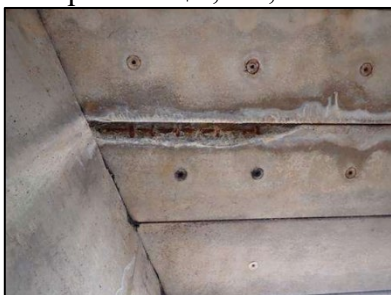
Images showing spalled concrete and exposed rebar at bridge joint on the underside of bridge and along curbline.
