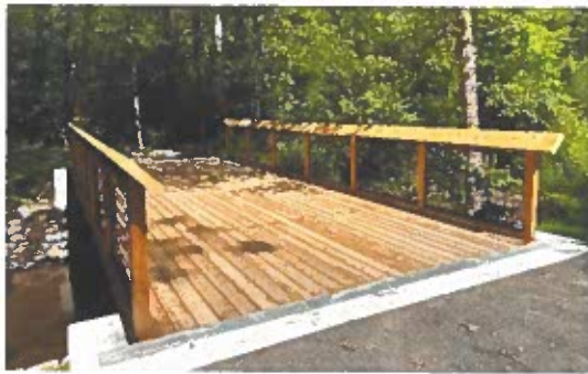
Westmoor Park Pedestrian Bridge Replacement
