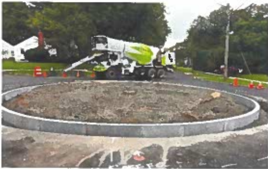
Roundabout Construction on King Philip Drive
