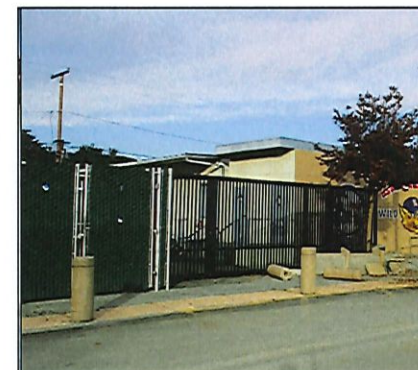
Security and Access Control
