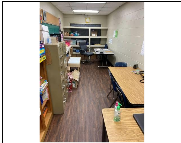
Photo #28. View of assumed ACBM dark wood looking LVT flooring in special education room #4.
