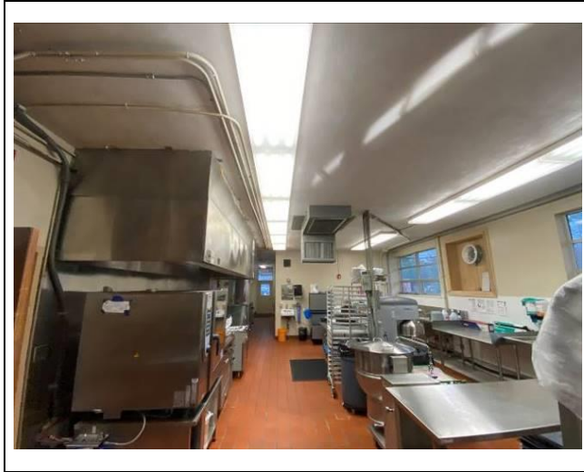
Photo #7. Another view of the kitchen in the original building.
