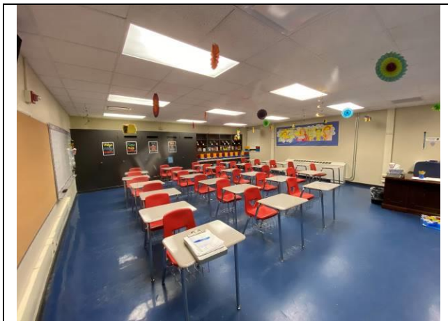
Photo #35. View of typical classroom found throughout the school.
