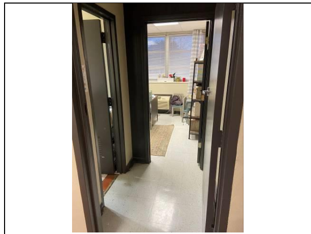
Photo #24. View of assumed ACBM whitish/gray (12"X12") floor tile with gray speckles in assistant principal office.
