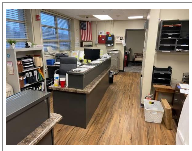
Photo #22. View of assumed ACBM light wood looking LVT flooring in office lobby area.
