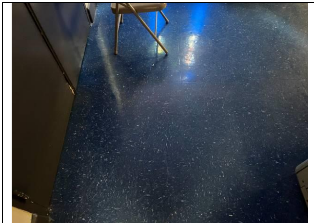
Photo #11. View of assumed dark blue with light blue speckles (12"X12") floor tile found in original bldg., 2 nd and 3 rd addition classrooms.
