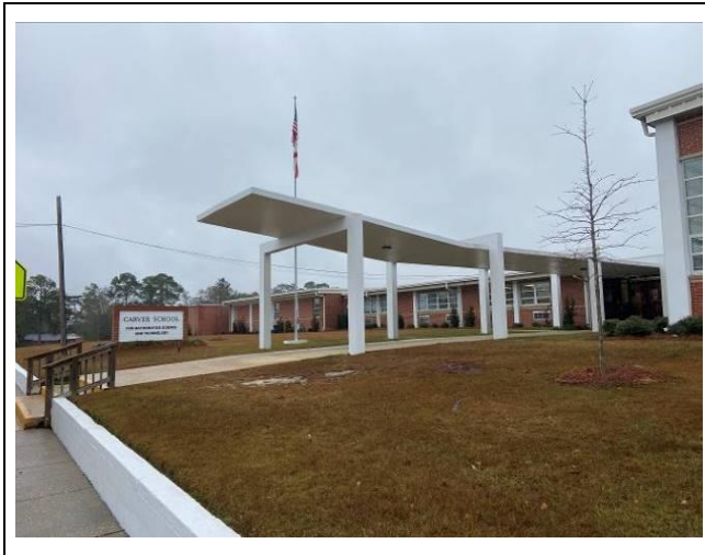
Photo #1. Typical Exterior Building Materials observed along main entrance to school.
