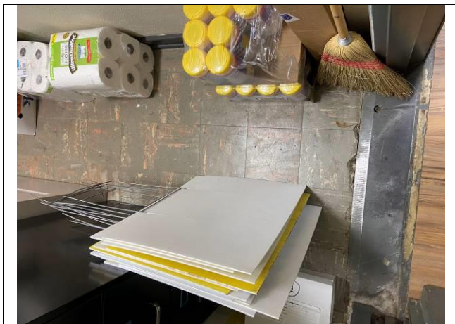
Photo #23. View of assumed ACBM greenish with white salmon streaks and gray/reddish (9"X9") floor tile in the safe in the office.
