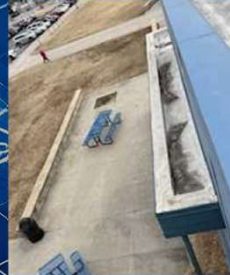
Replace canopy roof
