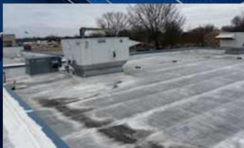
Install new cricket insulation behind each RTU Unit.
