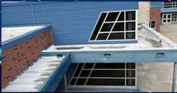
Replace flat roof canopy
