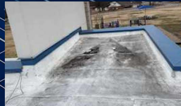
Replacing all counter flashing and coping cap.
