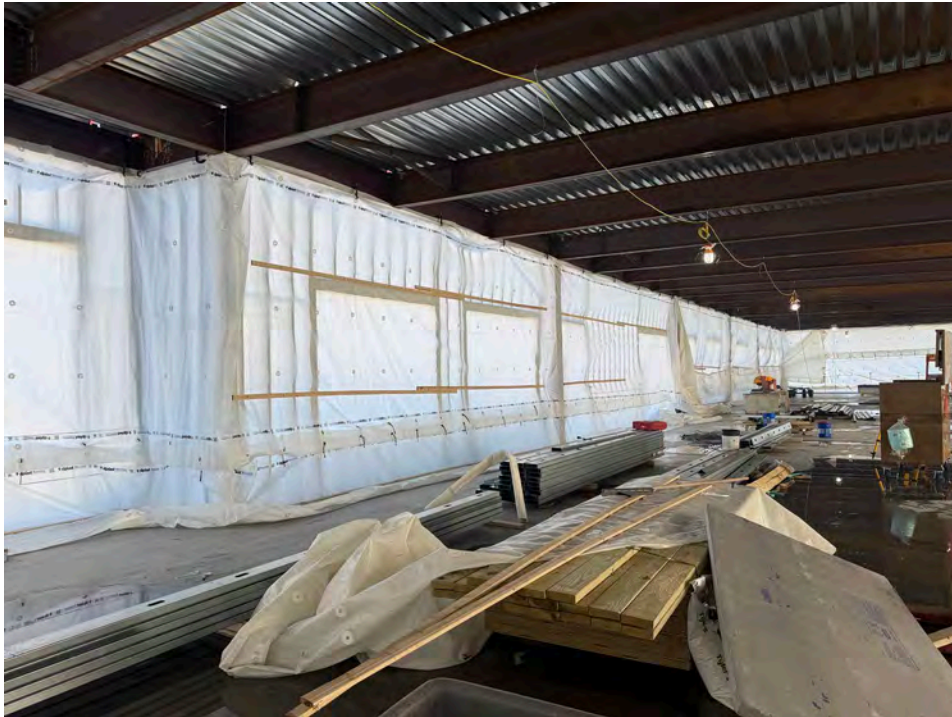
Feb. 27: Exterior Framing - Level 3
