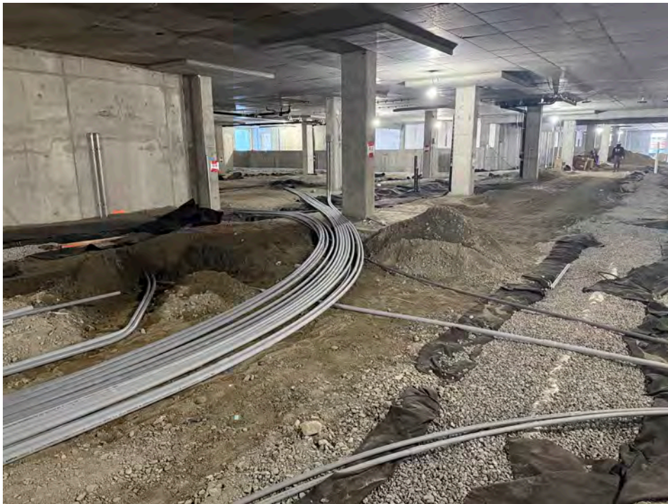
Feb. 26: Underground Utilities - Building A
