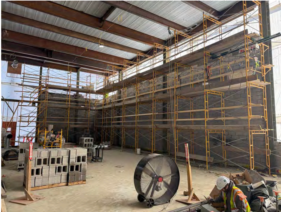
Feb. 19: CMU Progress - Gyms
