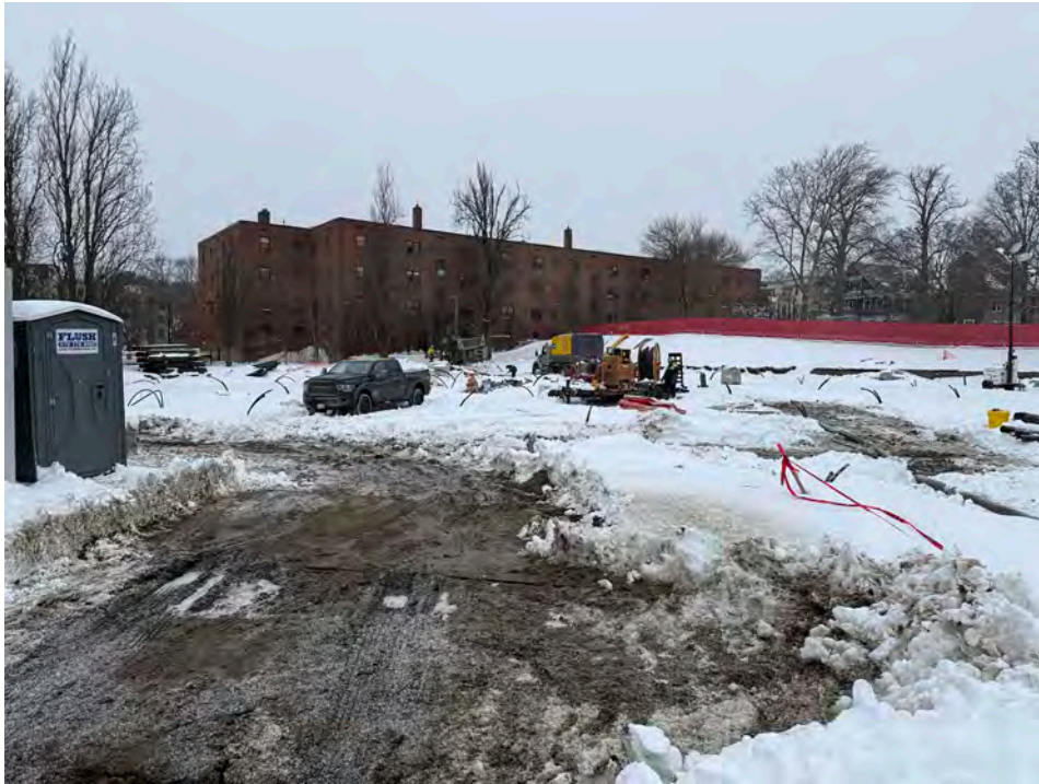
Feb. 25: Geothermal Well Drilling - Pierce Park
