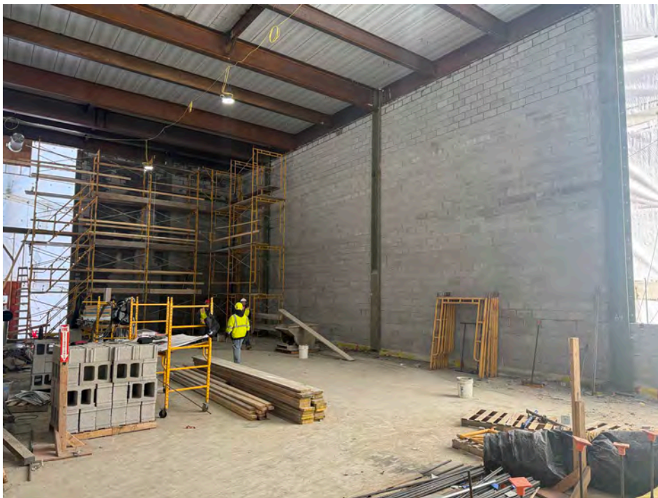
Feb. 27: CMU Progress - Gyms
