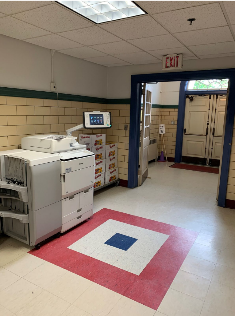
Hallways with copiers
