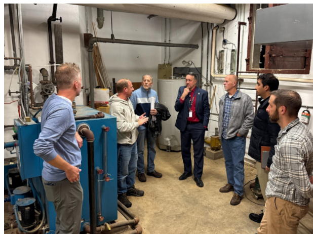
Community forum attendees seeing Falls-Lenox Primary School's boiler room, mechanical systems and crawl space first-hand.
