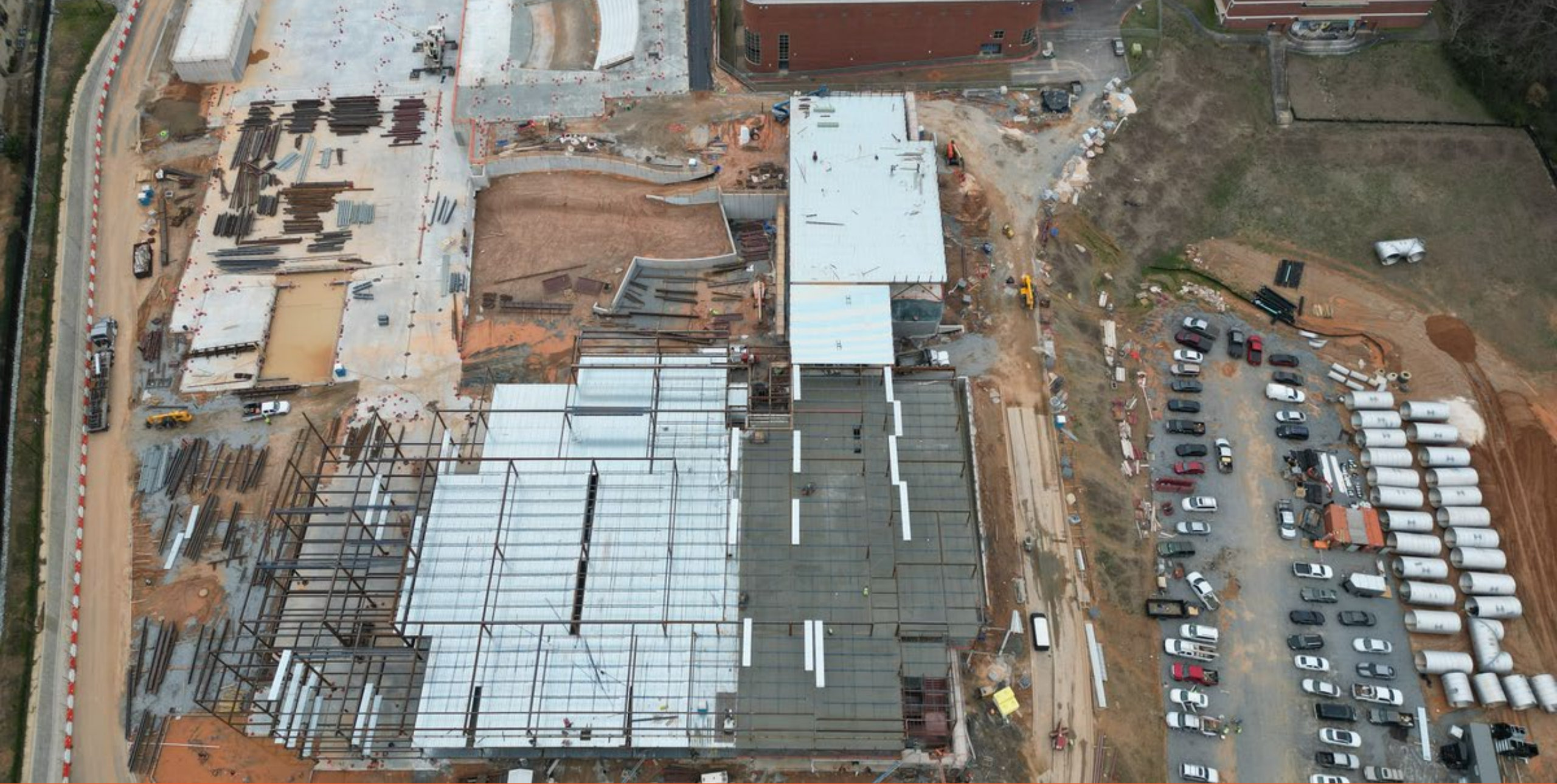
Overall Site Progress
