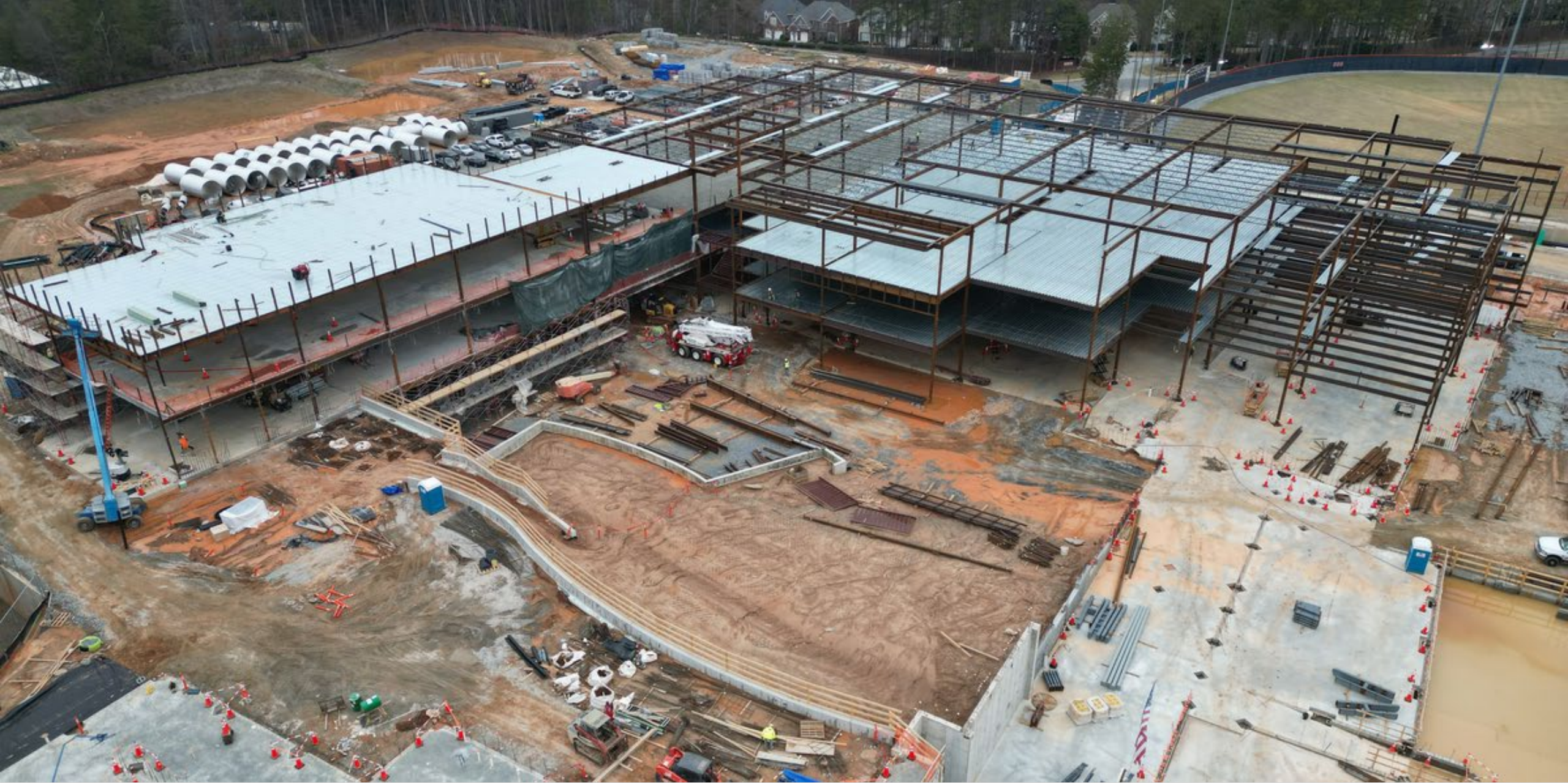
Overall Site Progress- View from South-West
