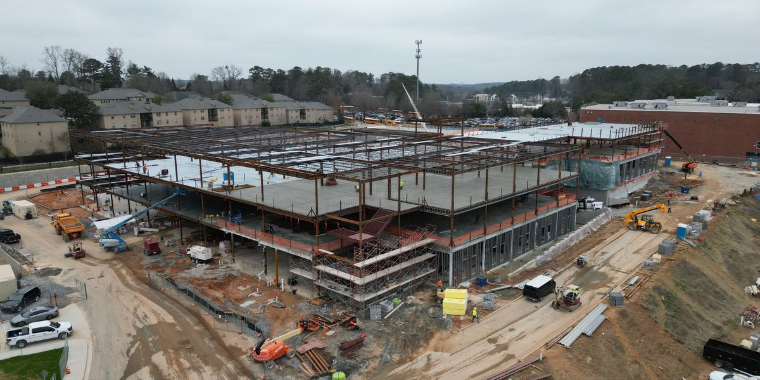
Site View from North-East- Area '2' and '3' Concrete Pour on all Levels.
