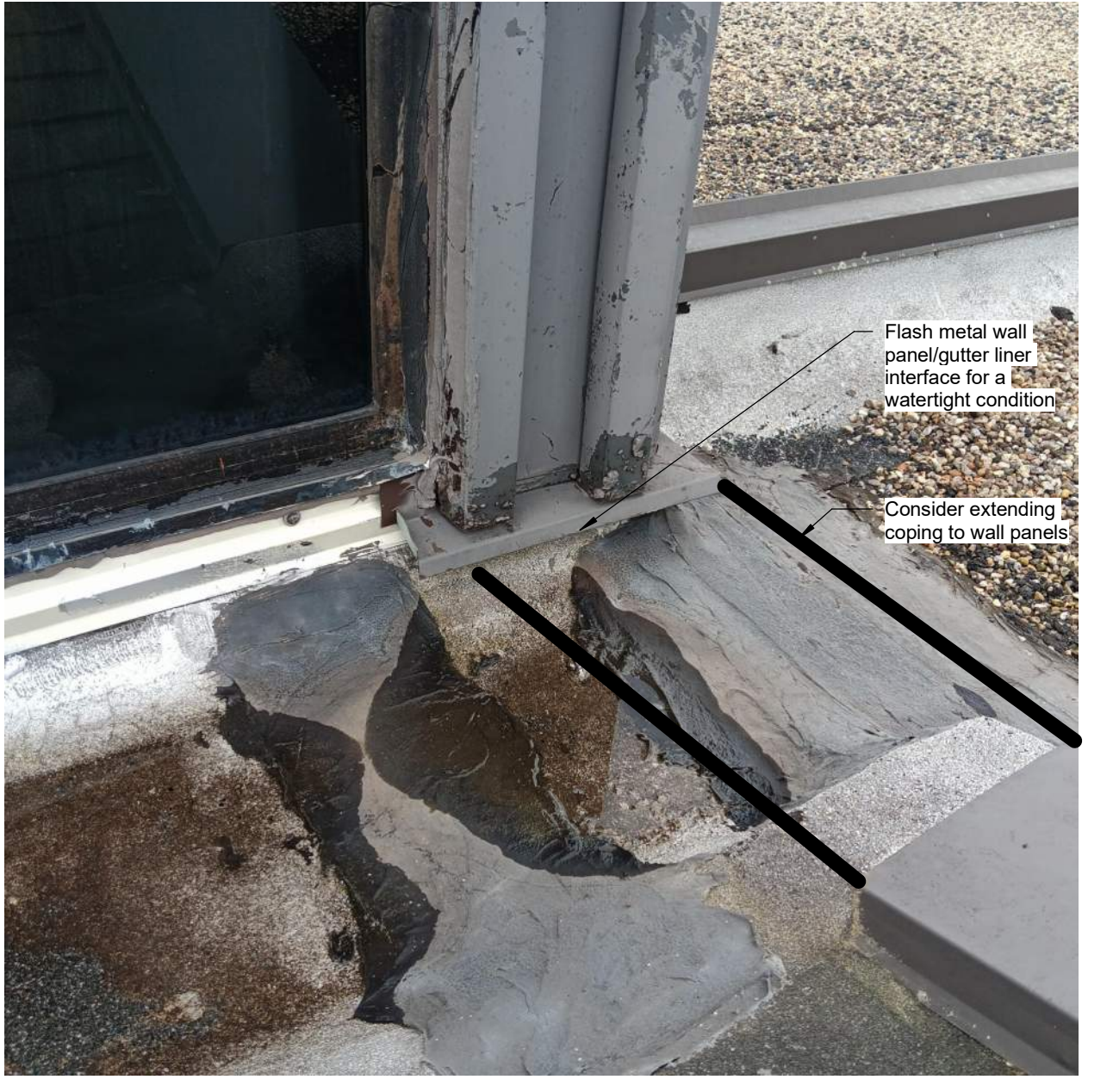
5 Gutter, Metal Siding, Coping, Roof Interface 1 1/2" = 1'-0"
