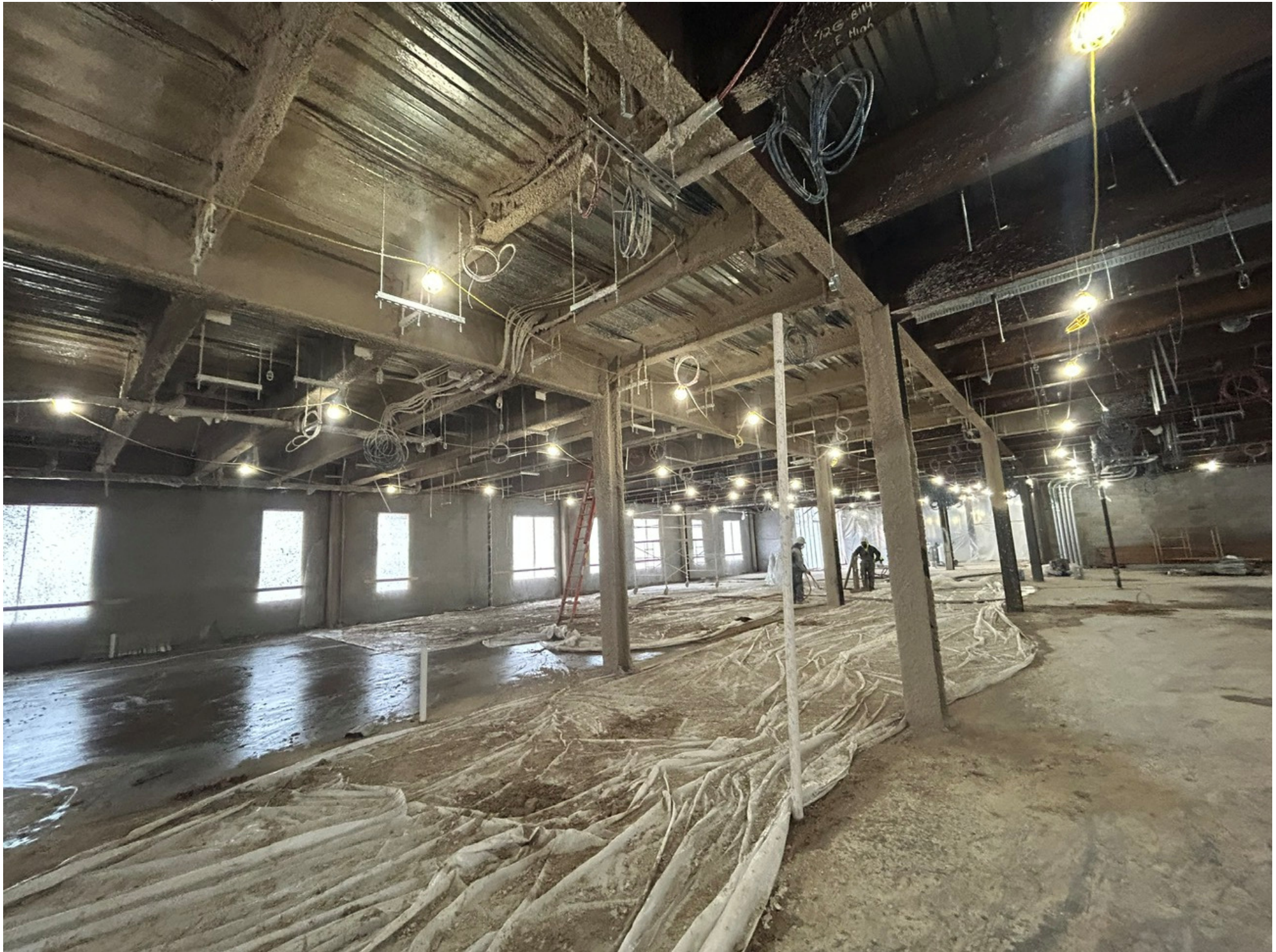
NORTH EAST MIDDLE / HIGH SCHOOL – REPLACEMENT – FIREPROOFING – HIGH SCHOOL WING – LEVEL 2
