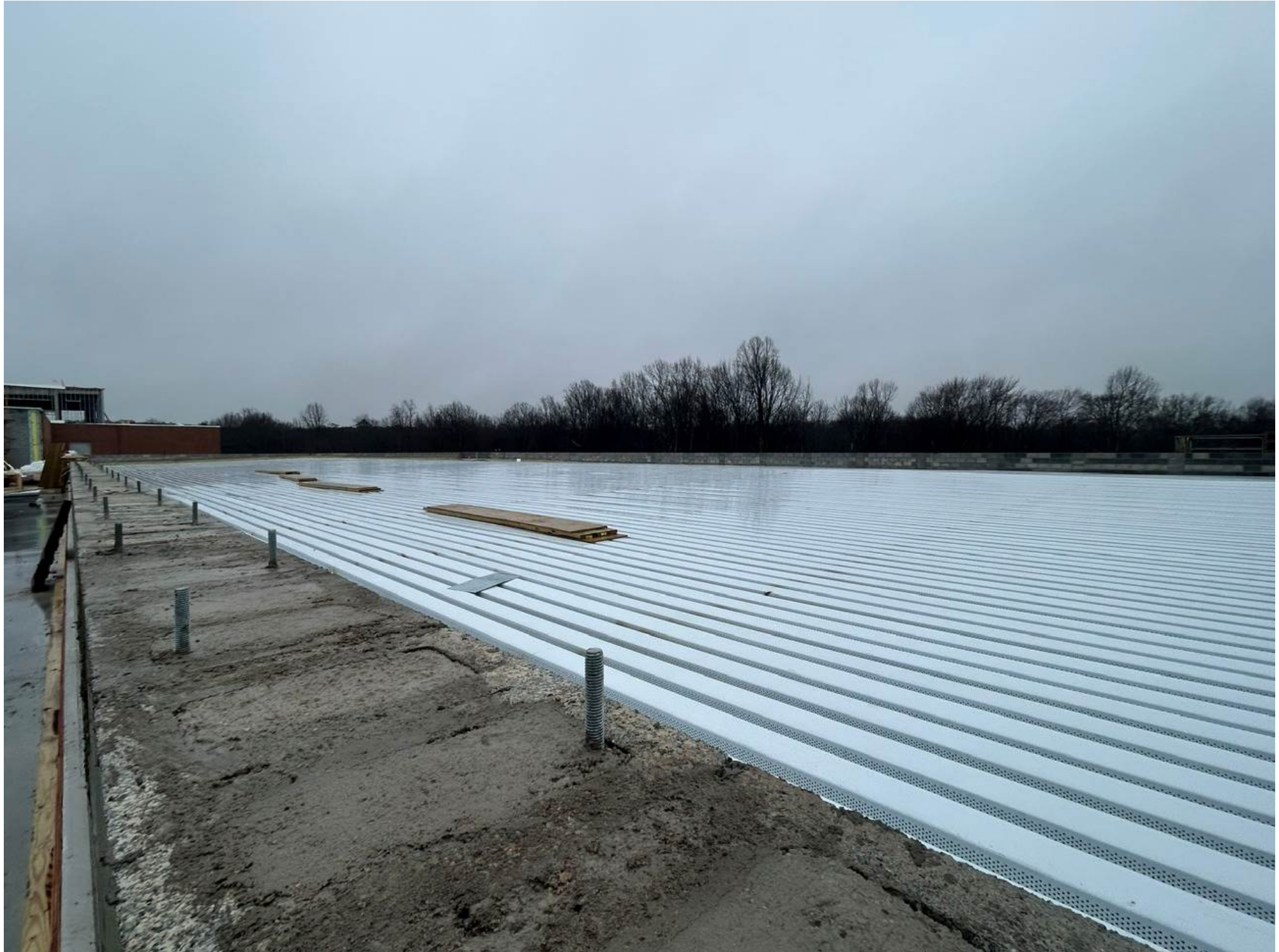
NORTH EAST MIDDLE / HIGH SCHOOL – REPLACEMENT – GYMNASIUM ROOF
