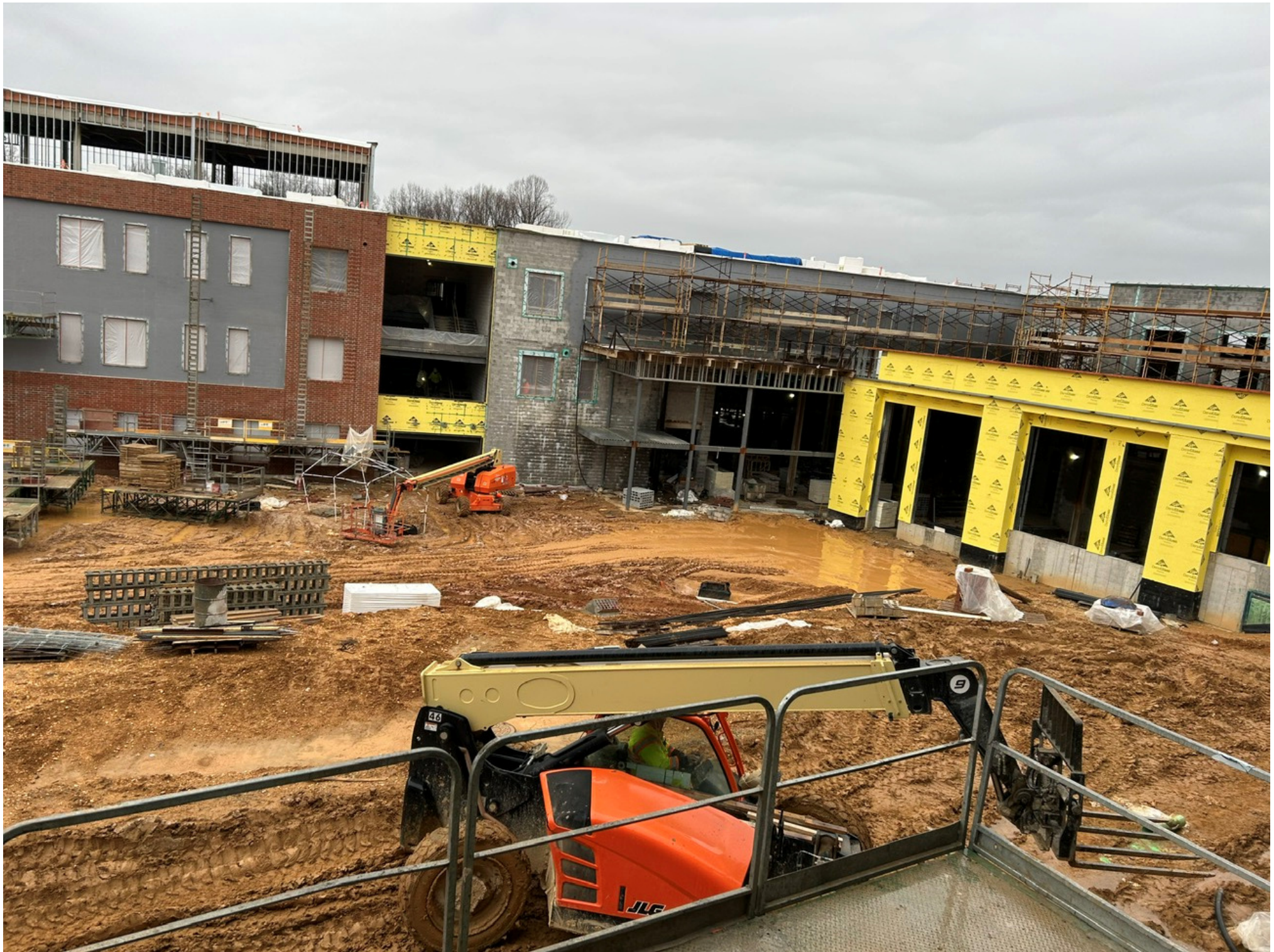
NORTH EAST MIDDLE / HIGH SCHOOL – REPLACEMENT – BRICK VENEER – MIDDLE SCHOOL WING/COURTYARD
