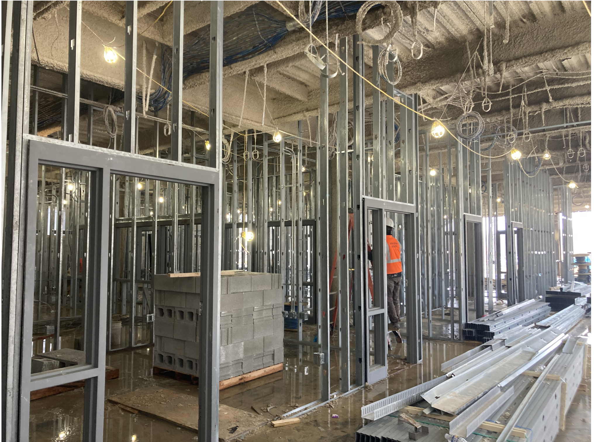
NORTH EAST MIDDLE / HIGH SCHOOL – REPLACEMENT – ADMINISTRATION WING – FRAMING
