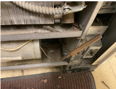
Capillary Tube.v2.jpg; Added on 6/15/2023 9:42:09 PM by danhainey@cm3inc.com
