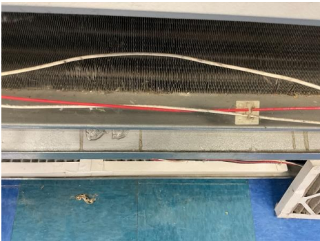
Wiring.v2.jpg; Added on 6/13/2023 5:03:52 PM by danhaihey@cm3inc.com
