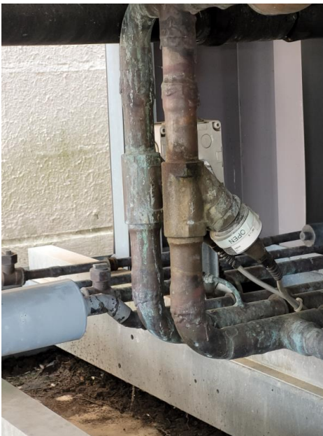
HotGasBypass.v2.jpg; Added on 5/24/2023 10:47:53 AM by danhainey@cm3inc.com
