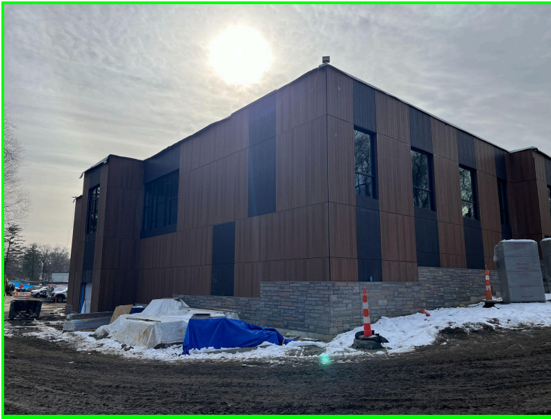
Photo 1: Exterior façade installation ongoing, south-east corner
