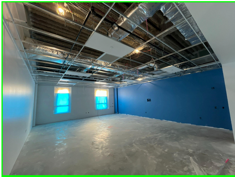
Photo 2: Painted classroom space with flooring installed
