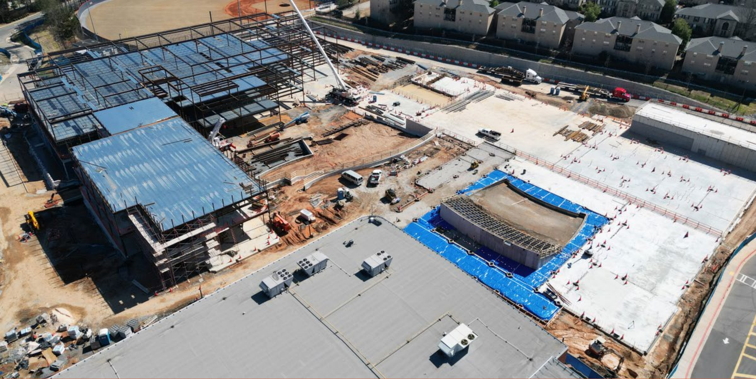
Overall Site Progress- View from North-West
