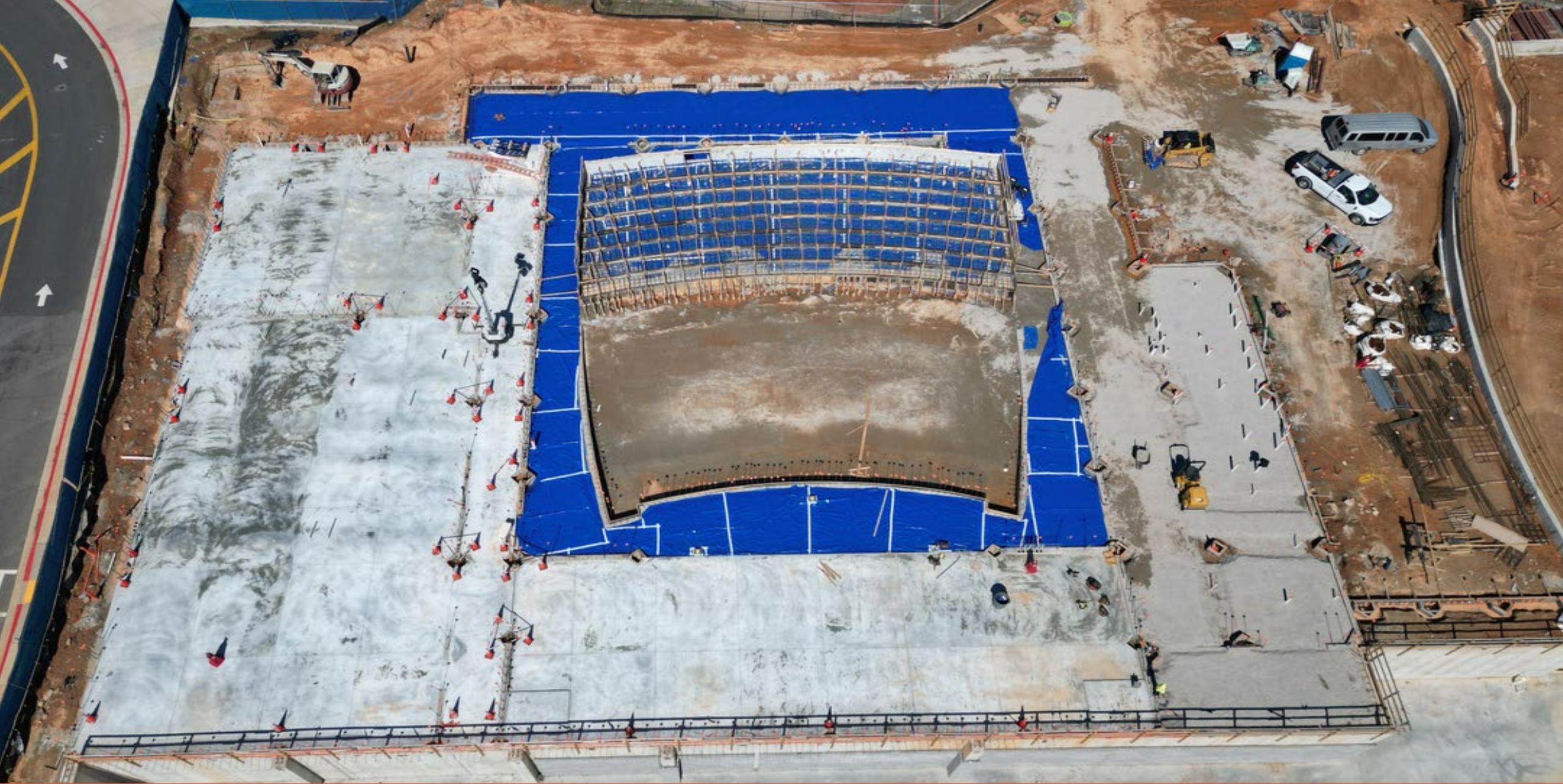
Auditorium (Area 8) in progress
