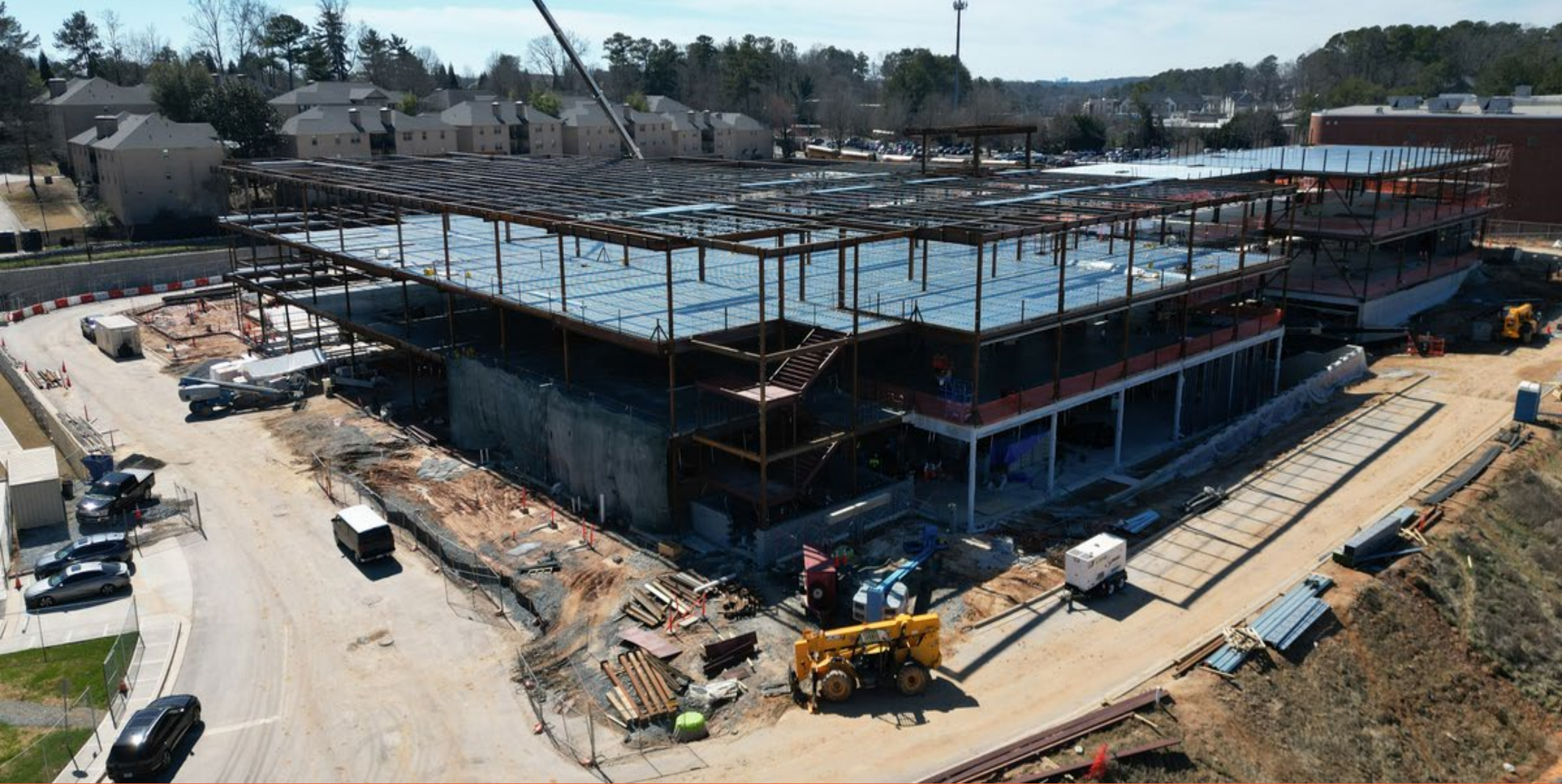
Area 2, 3 and 4 Steel Erection, Staircase and Exterior CMU
