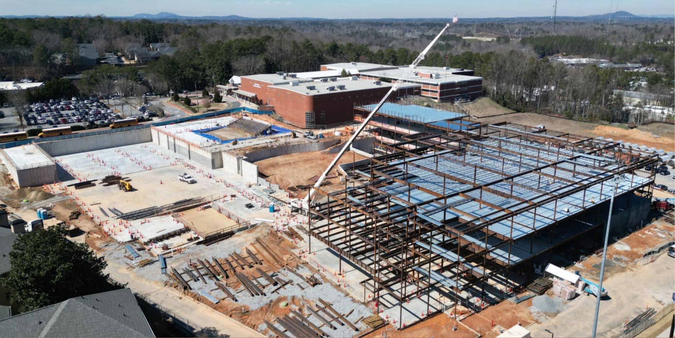
Overall Site Progress- View from South-East
