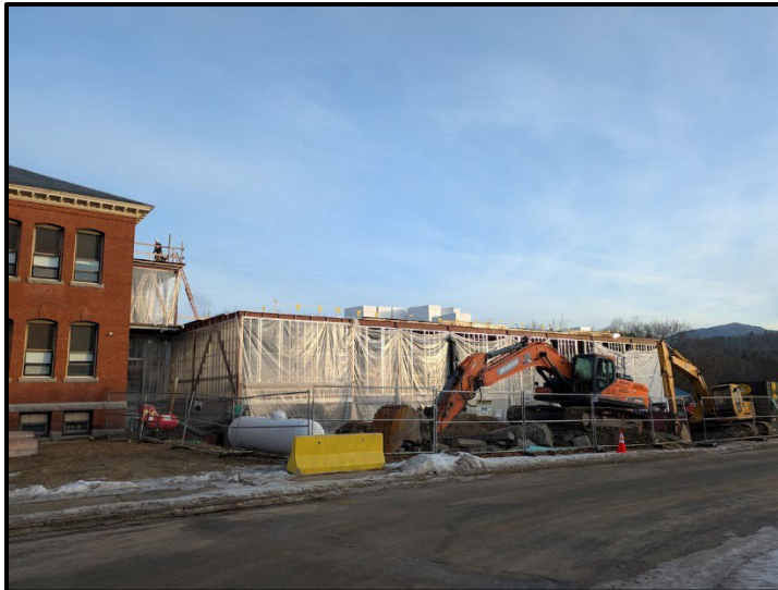
Work at Troy Elementary School 1/14/2026. Photo courtesy of Andrew Dey.
