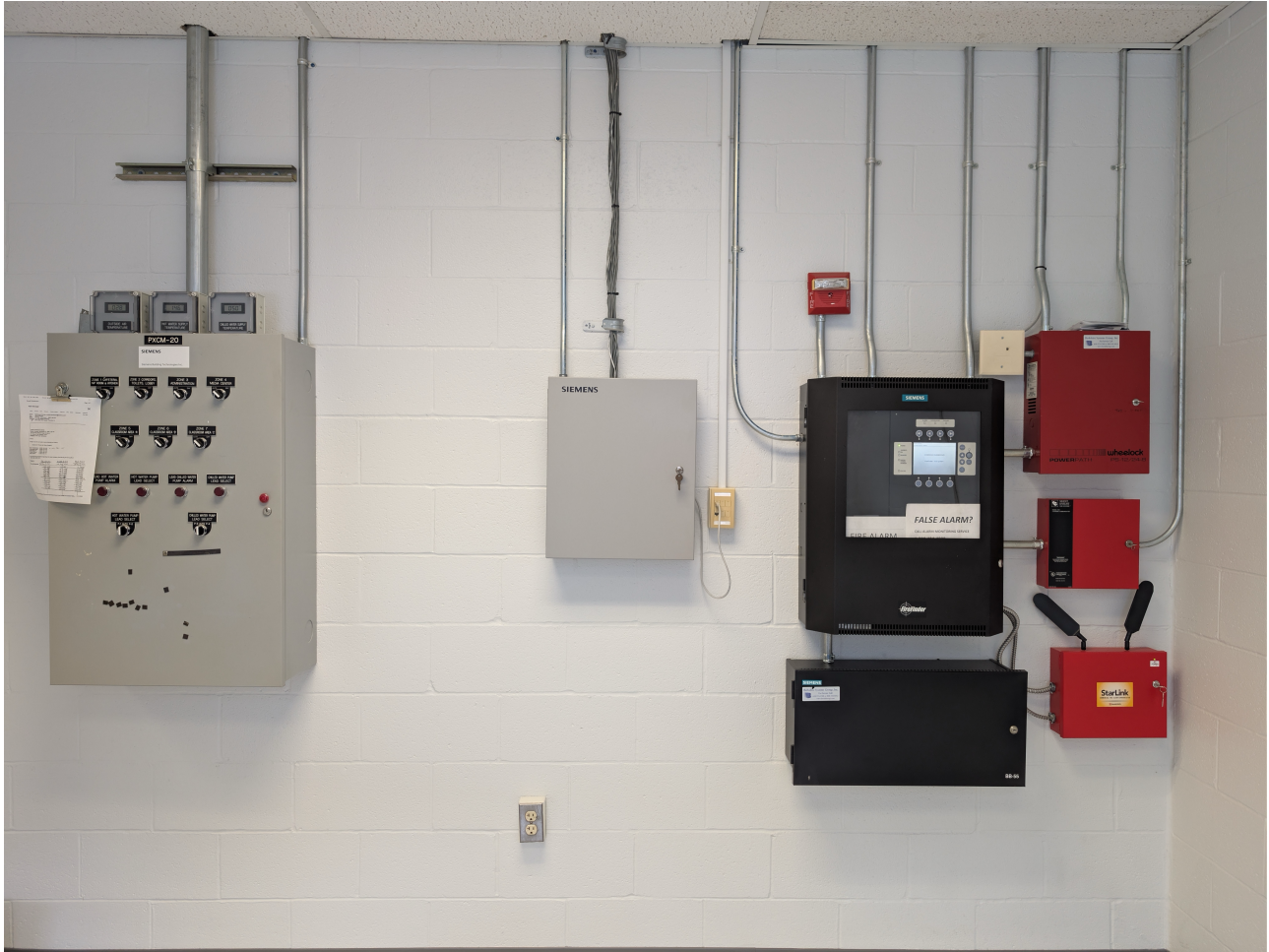
Existing Equipment in IPC Room Where CMU Wall To Be Demolished
