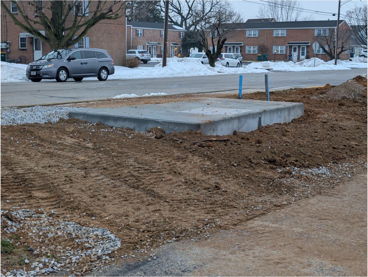
New Water Meter Pit Installed
