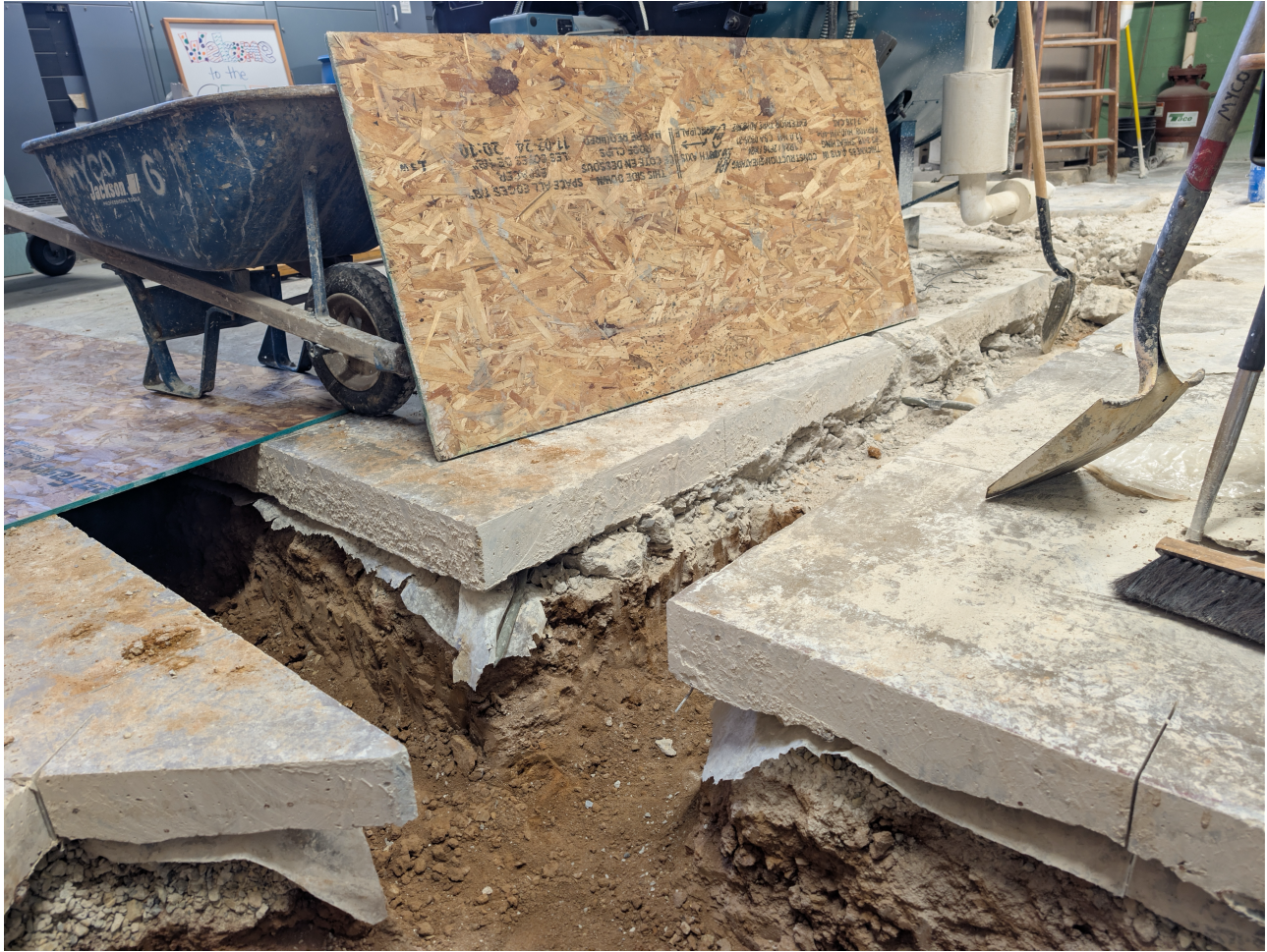
Excavation in West Boiler Room for New Plumbing
