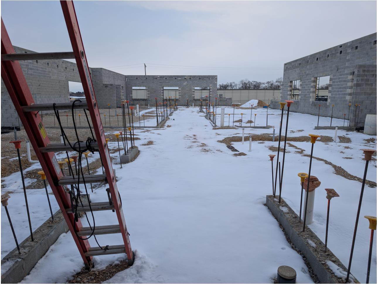
Current Condition North Wing Area D
