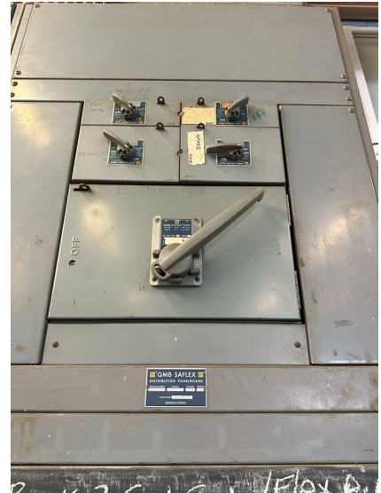
Figure 11: Service Switchboard with Spare Switches
