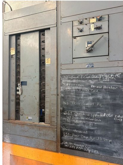
Figure 10: 1600A Service Equipment in Building
