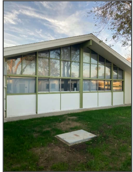
Building A Exterior
