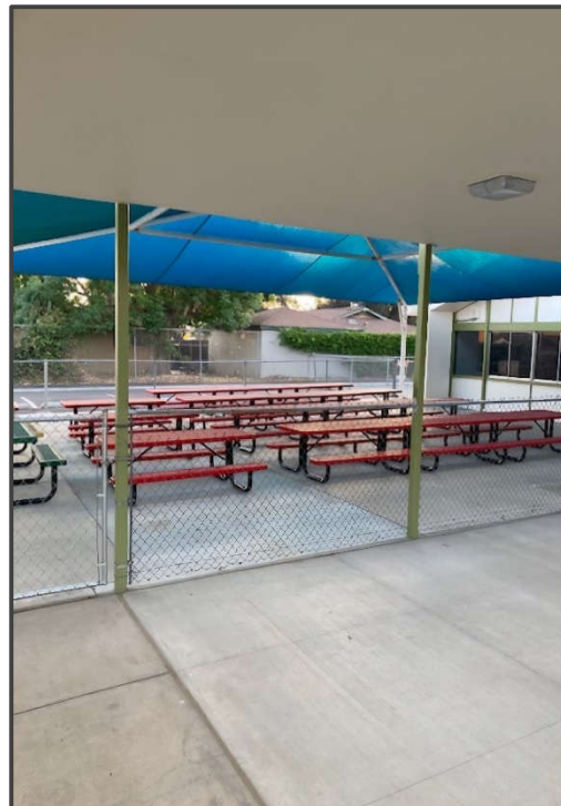
New Electrical Service
