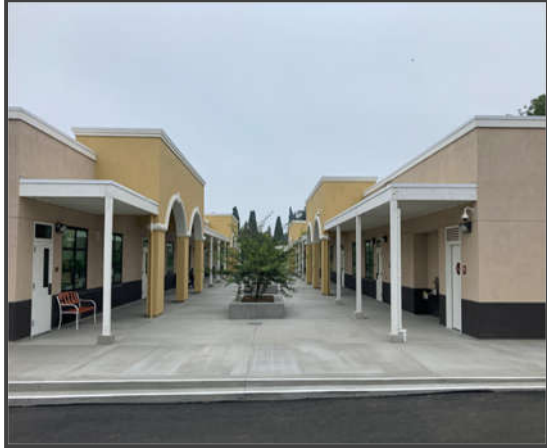
New Classroom Buildings
