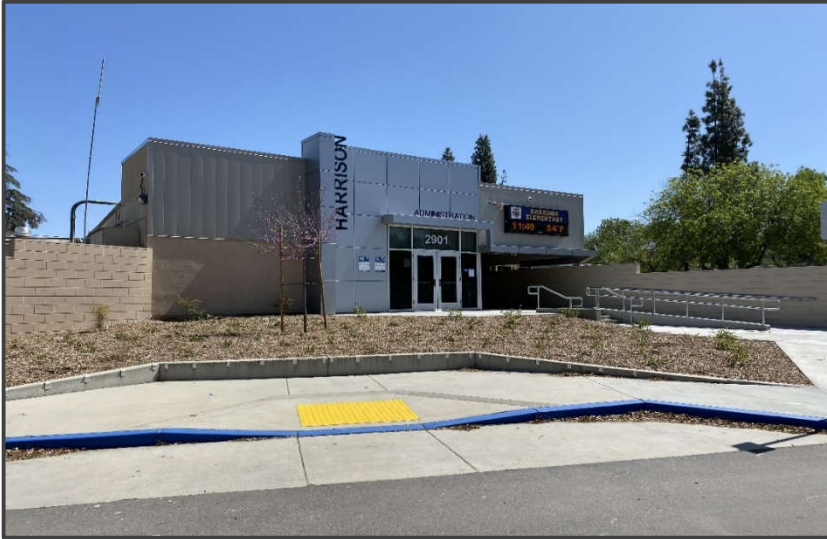
Completed Administration Building
