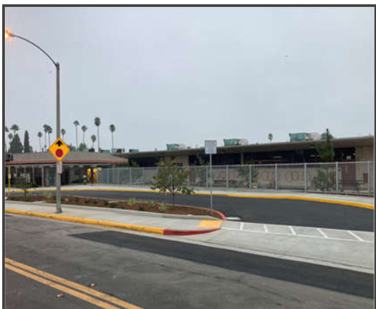
New Drop Off Area
