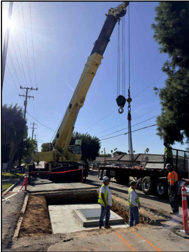
Increment 1 – Park Ave. Electrical Vault Craning
