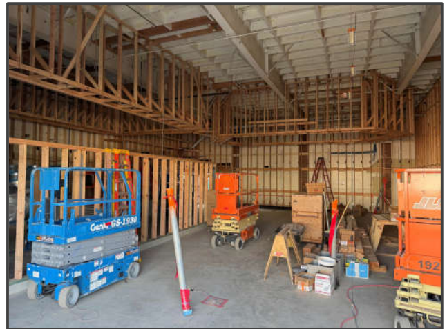
CTE – In-Wall Plumbing Work
