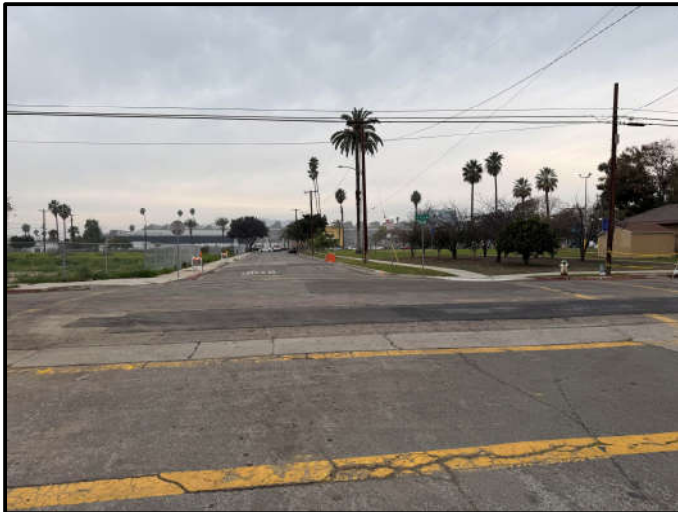
Increment 1 – 13 th St. Asphalt Patch
