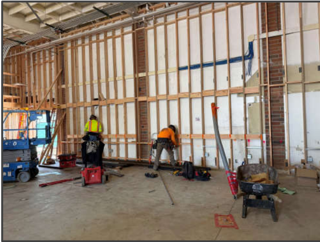
CTE – In-Wall Electrical Work
