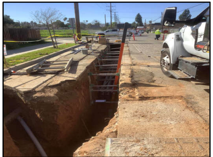
Increment 1 – Park Ave. Electrical Trench & Infrastructure Installation
