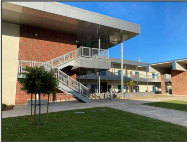
New 2-Story Classroom Building
