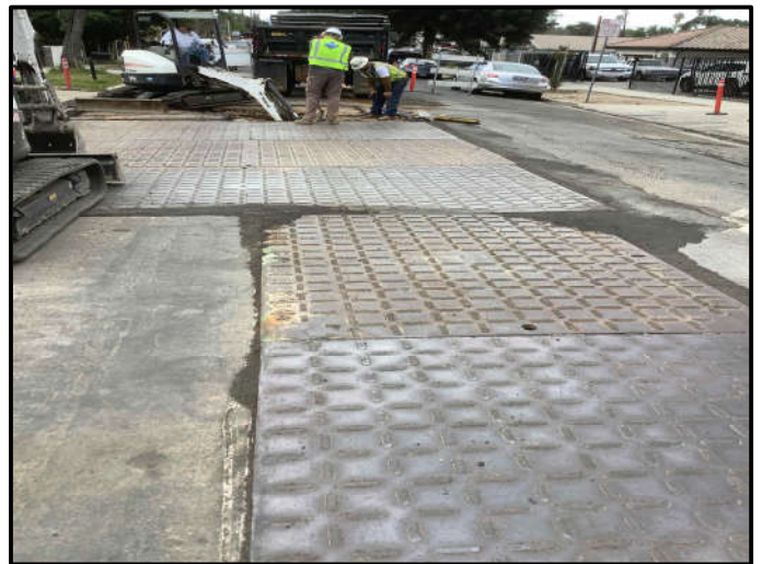
Increment 1 – Park Ave. Electrical Trenching
