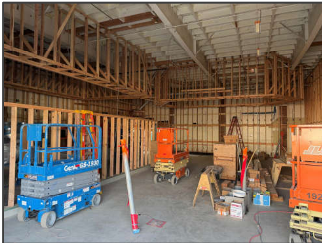
CTE – Wall Framing & In-Wall MEP Infrastructure Work
