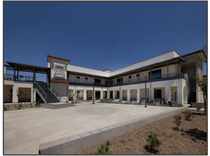
Building F – 2 Story Classroom
