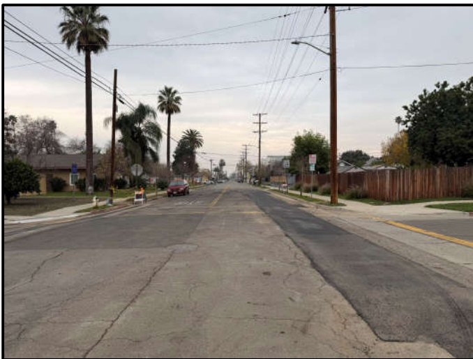
Increment 1 – Park Ave. Asphalt Patch
