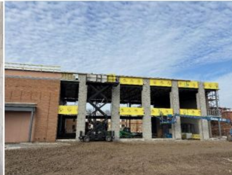
Area F Exterior Enclosure
