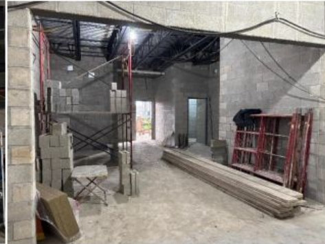
Area G Interior Masonry
