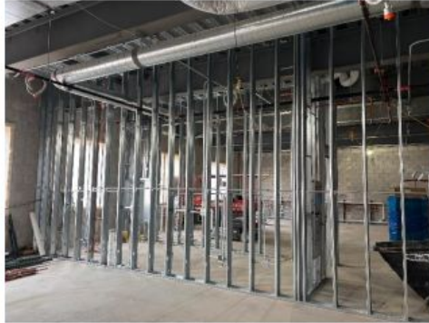
Area B 1 st Floor Framing
