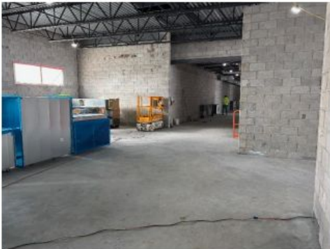
Area B/G 2 nd Floor Slab
