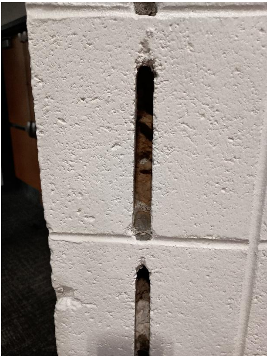
Figure 5. Current painted acoustic CMU
