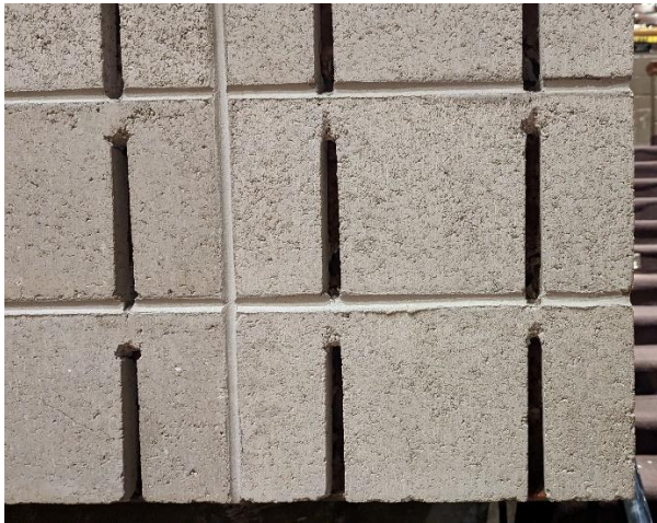
Figure 2. Pre-renovation unpainted acoustic CMU
