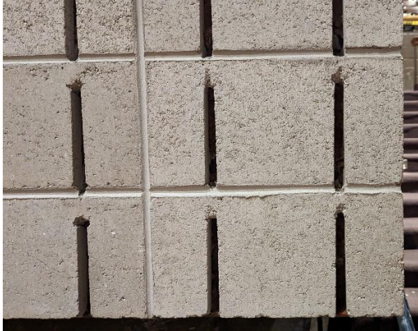
Figure 2. Existing acoustic CMU
