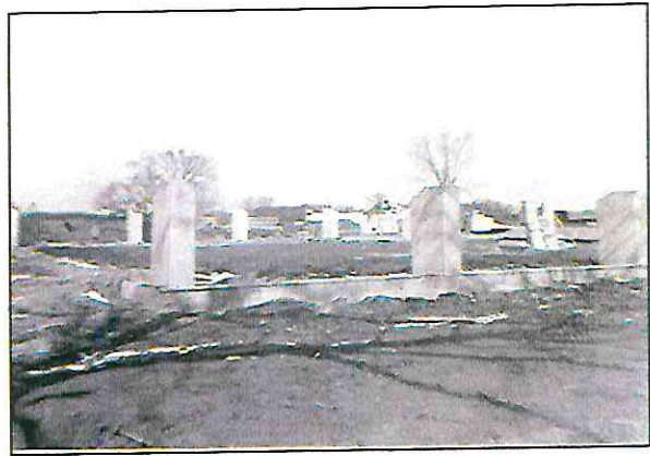
Byron gym under construction 1955
