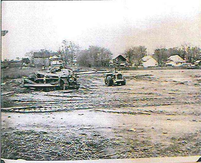
Working on ground south of New High School.
