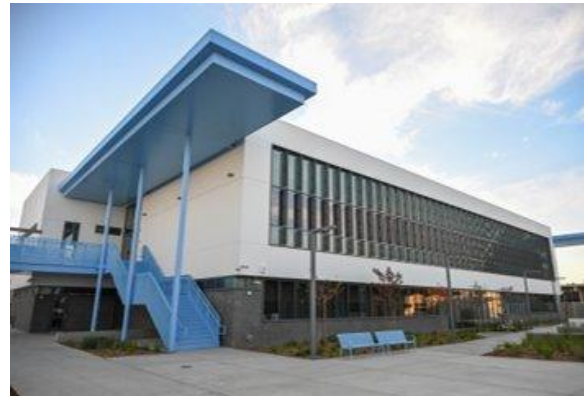
New Two-Story Classroom
