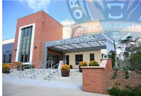
New Two-Story Classroom and Administration Building
