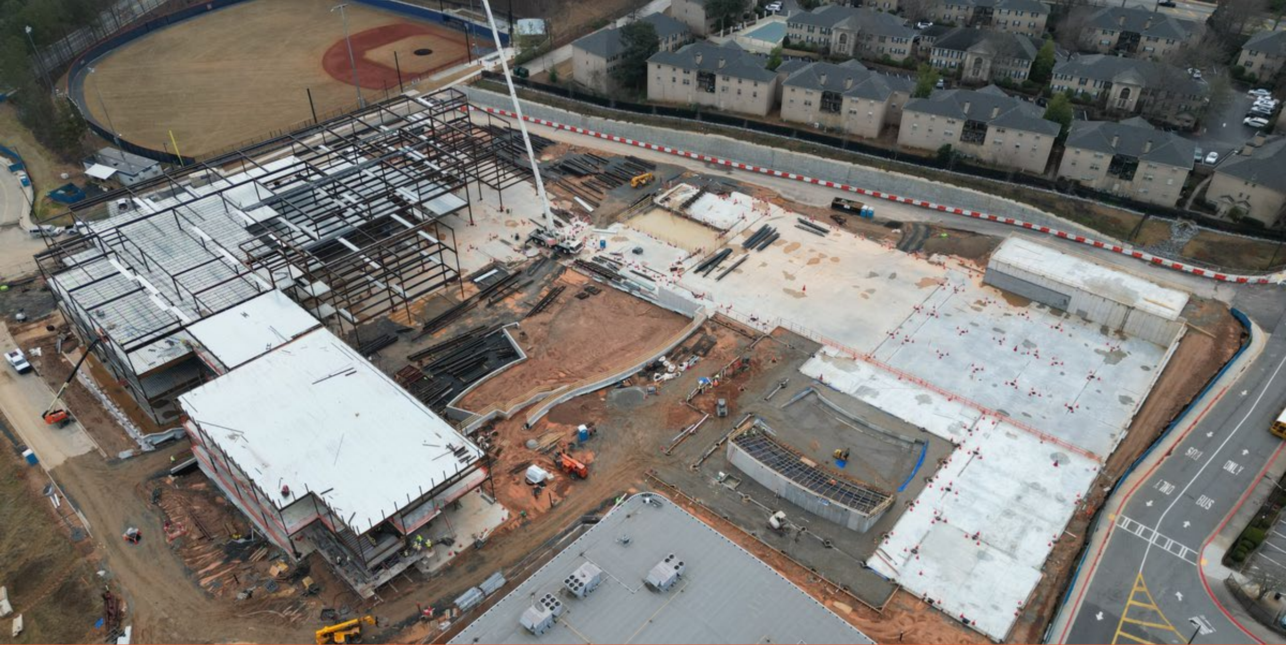
Overall Site Progress- View from North-West
