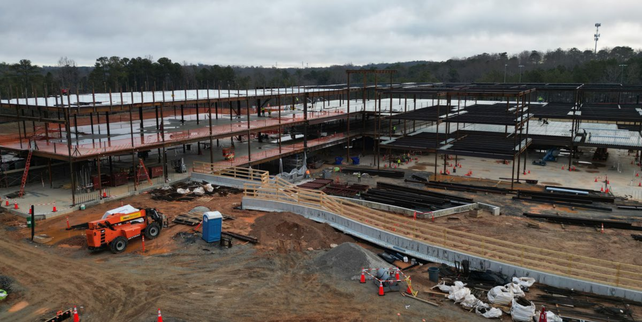
Courtyard retaining walls and Steel Erection progress.
