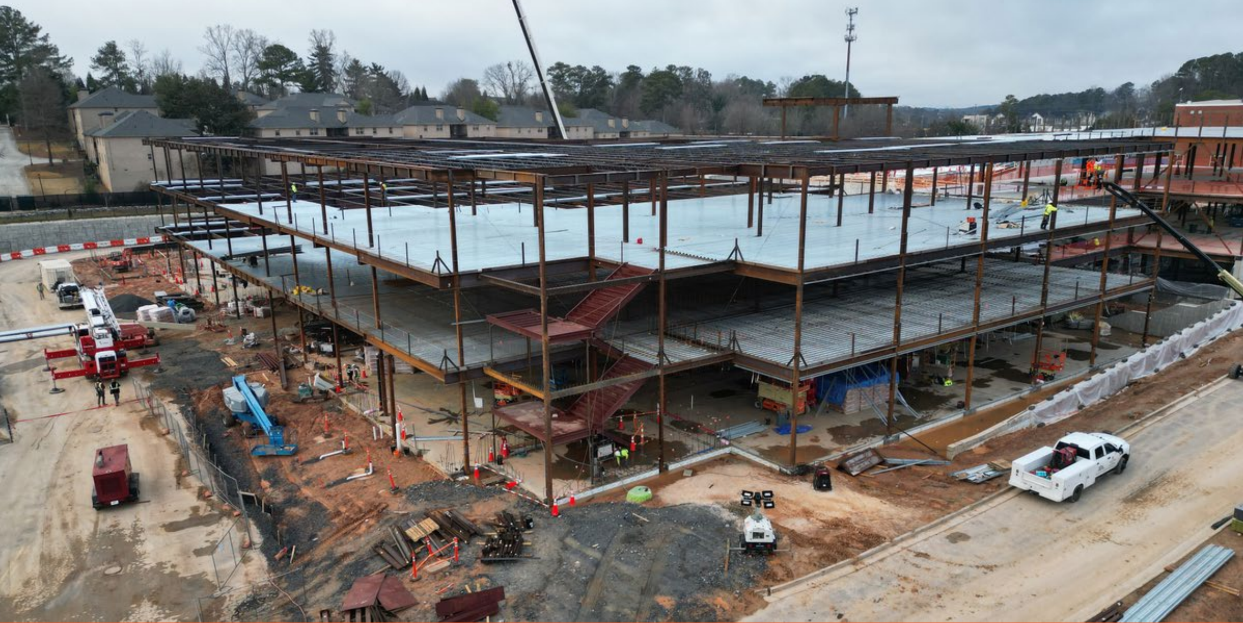
Area '3' Level 2 and 3 Elevated Slab Pour and Staircase
