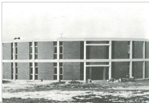
addition, as seen from the relocated hockey rink, gives evidence of the school dis-
