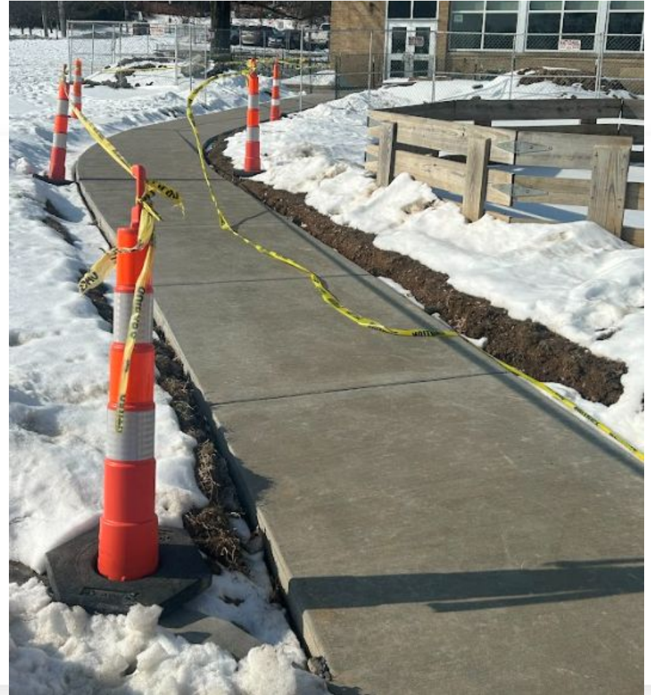
Hixson Sidewalk Replacement
