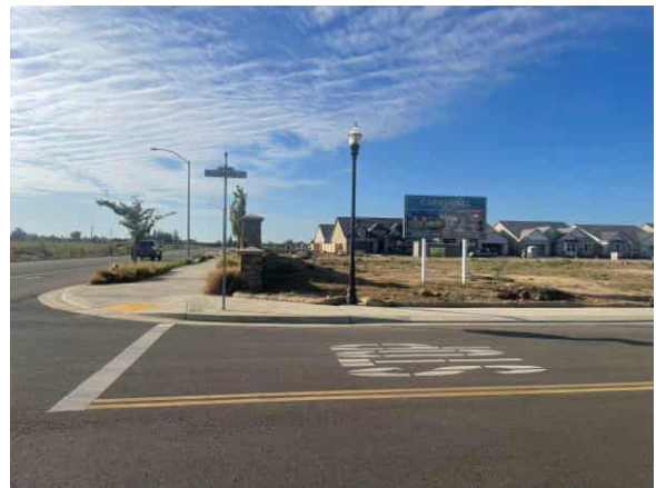
Photo #12 View of the western adjoining housing development.
