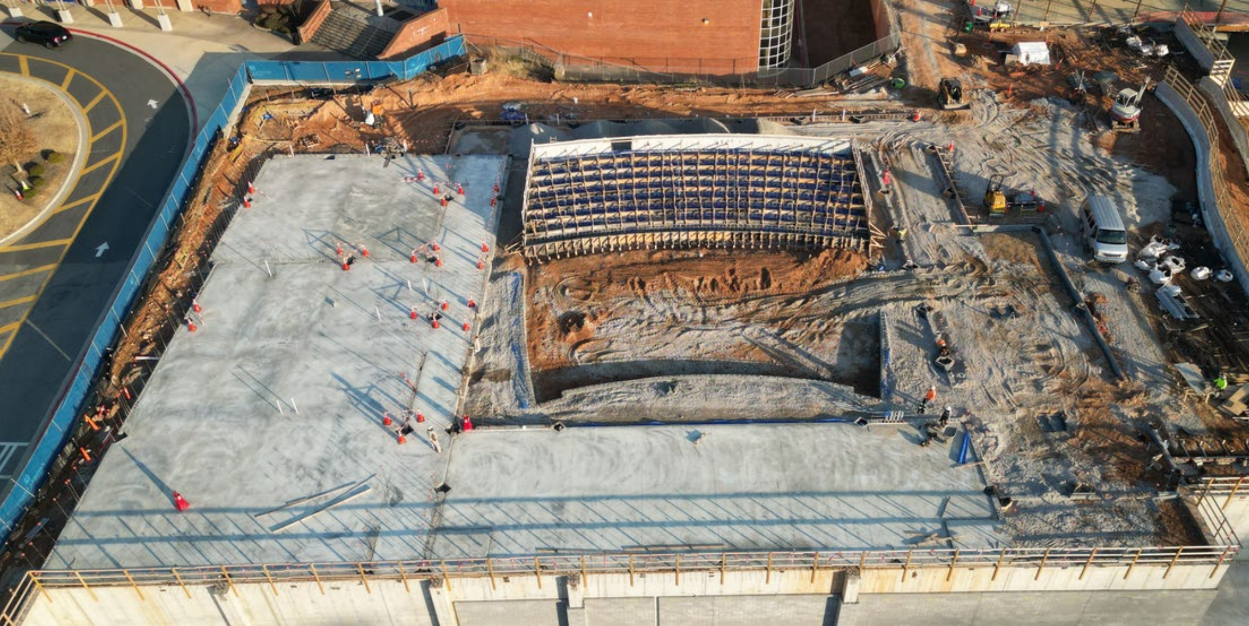
Main Building- Area 8 (Auditorium) in progress.
