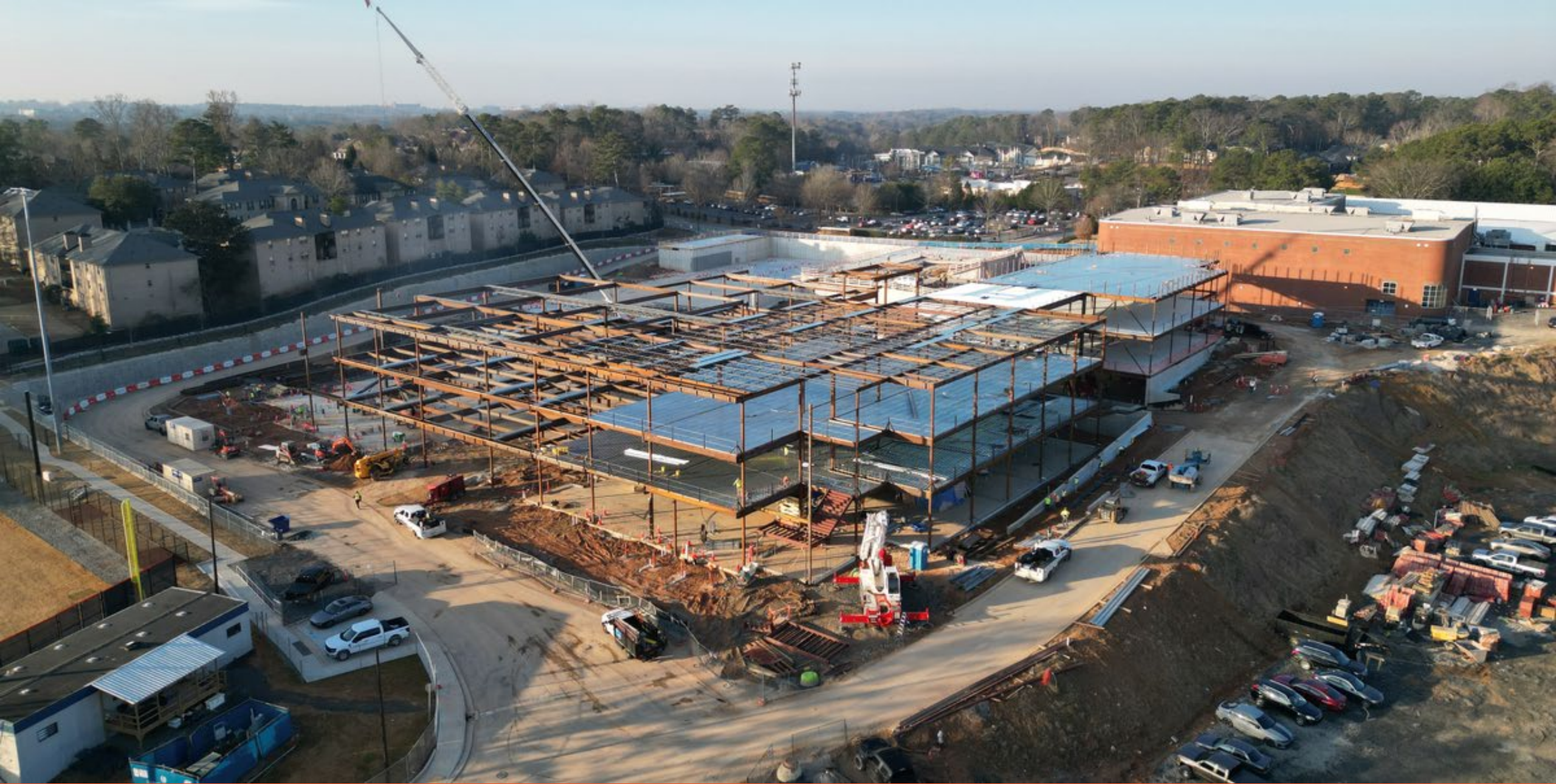
Overall Site Progress- Aerial View from South-East
