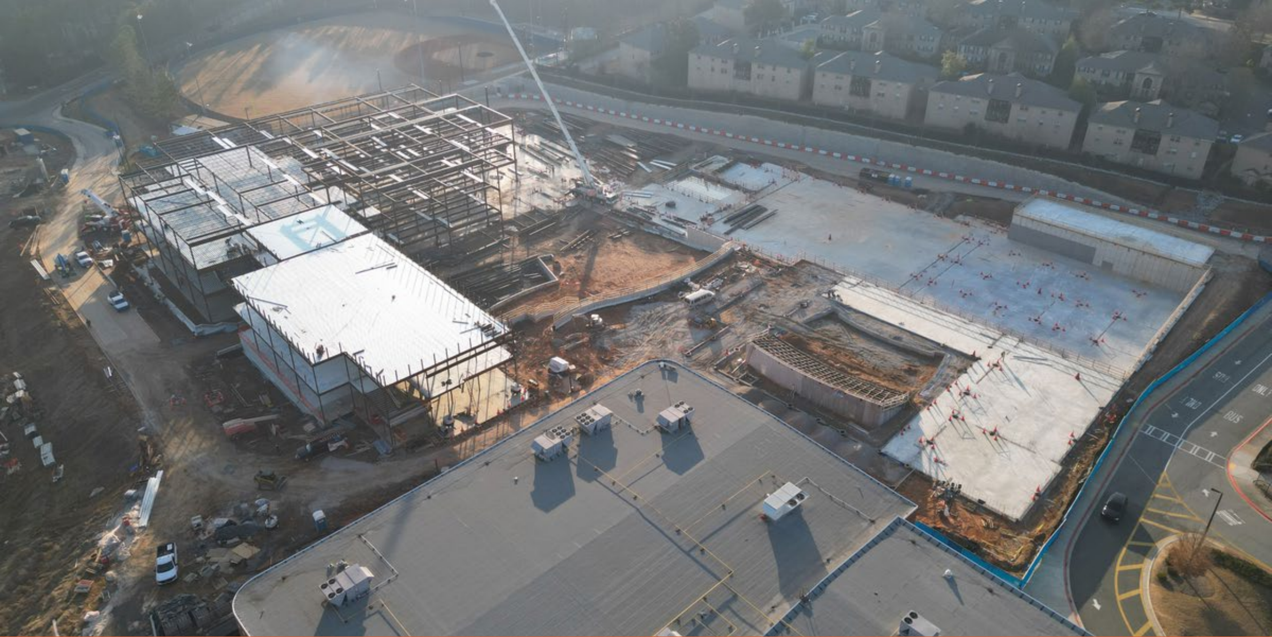
Overall Site Progress- Aerial view from North-West
