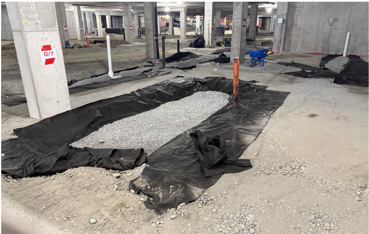
Underground Plumbing Backfilled, Garage Level Building A
