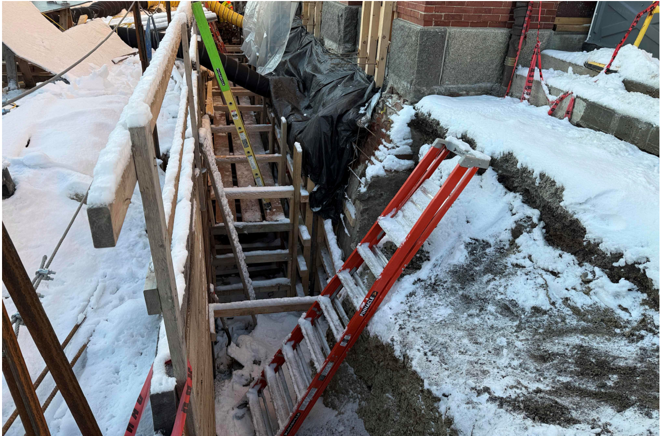
Heating Forms Ahead of Concrete Placement
