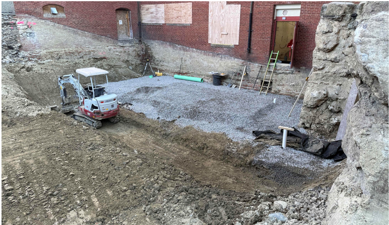
Foundation Excavation at Historic Building
