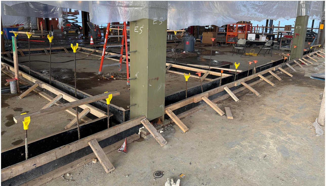
Forms for Curbs, L1 Building A
