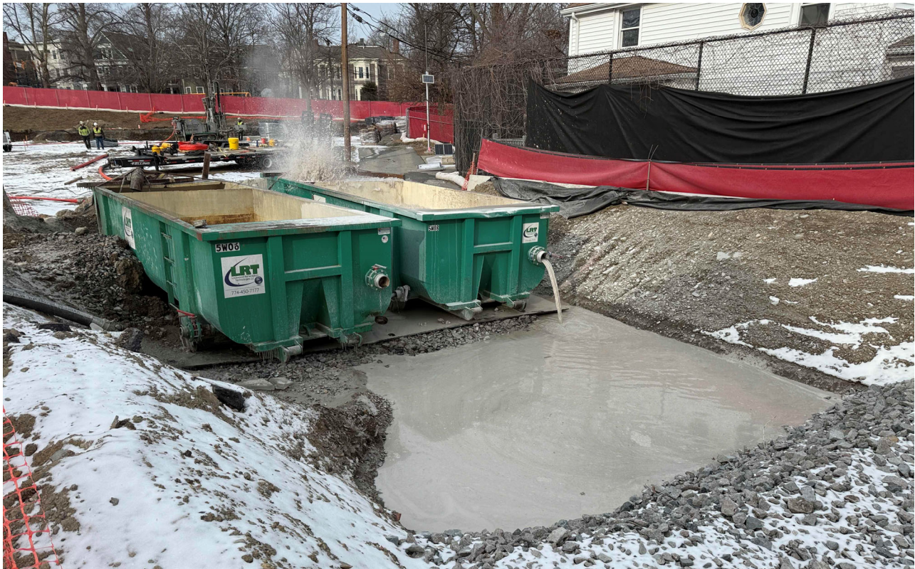
Water management, Pierce Park Geothermal Well Drilling
