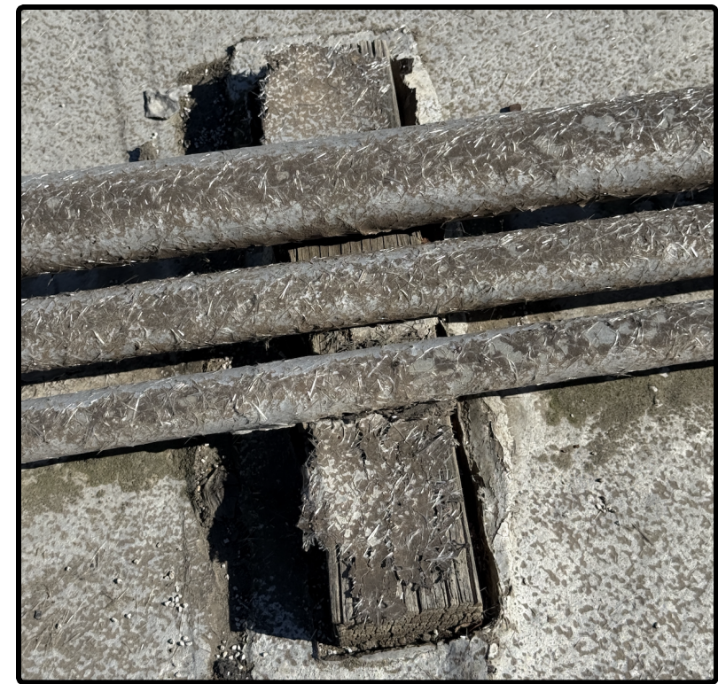
Wood pipe support blocks have damaged the silver emulsion coating and BUR membrane.
