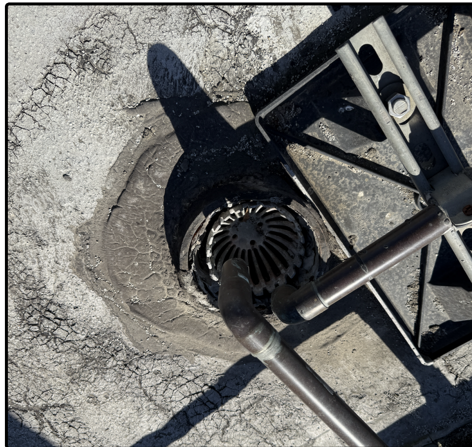
Membrane around condensate drain is cracked and deteriorated.
