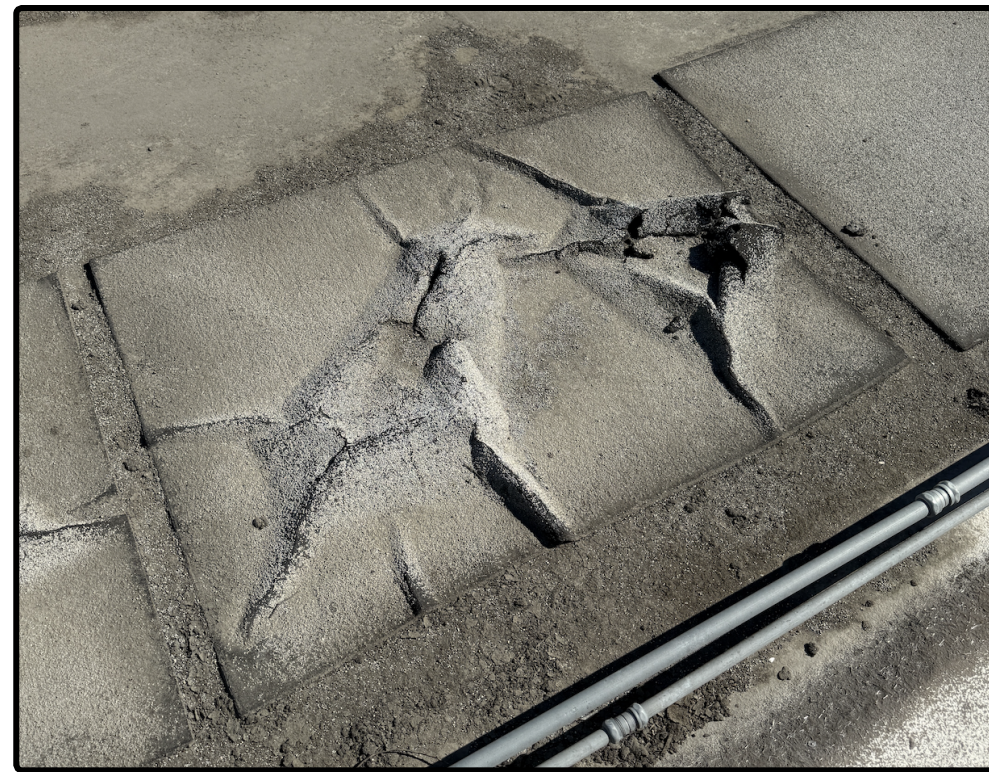
Walkway pads are severely blistered and deteriorated.
