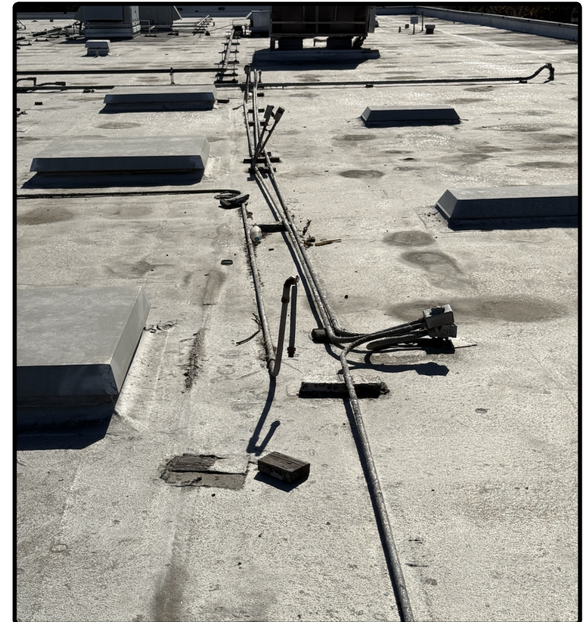
Several abandoned conduits and curbs, to be removed during reroof project
