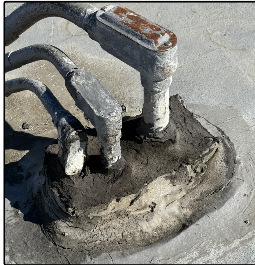
Conduit penetration flashings are brittle and cracking. Mastic is separating from the membrane
