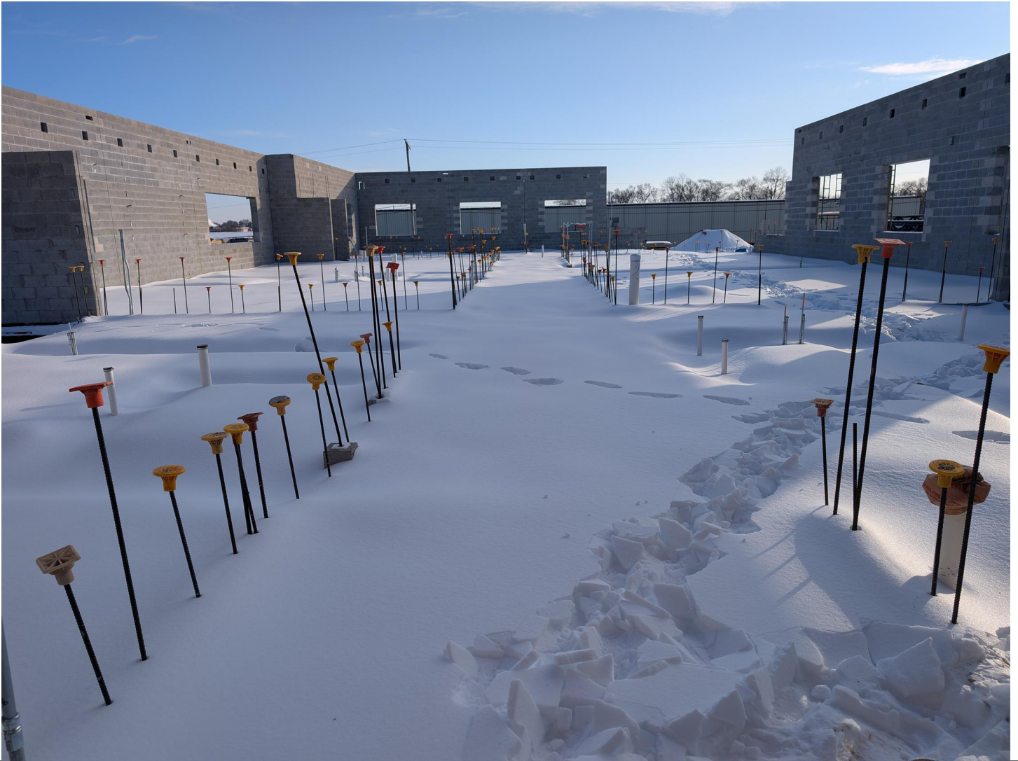
Current State of classroom addition wing
