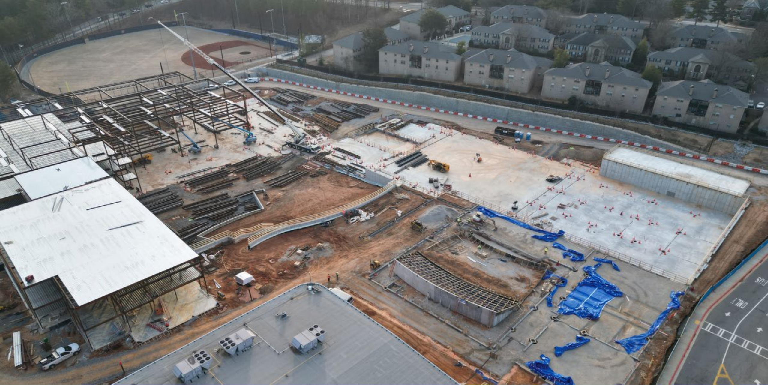
Overall Site Progress- Aerial view from North-West
