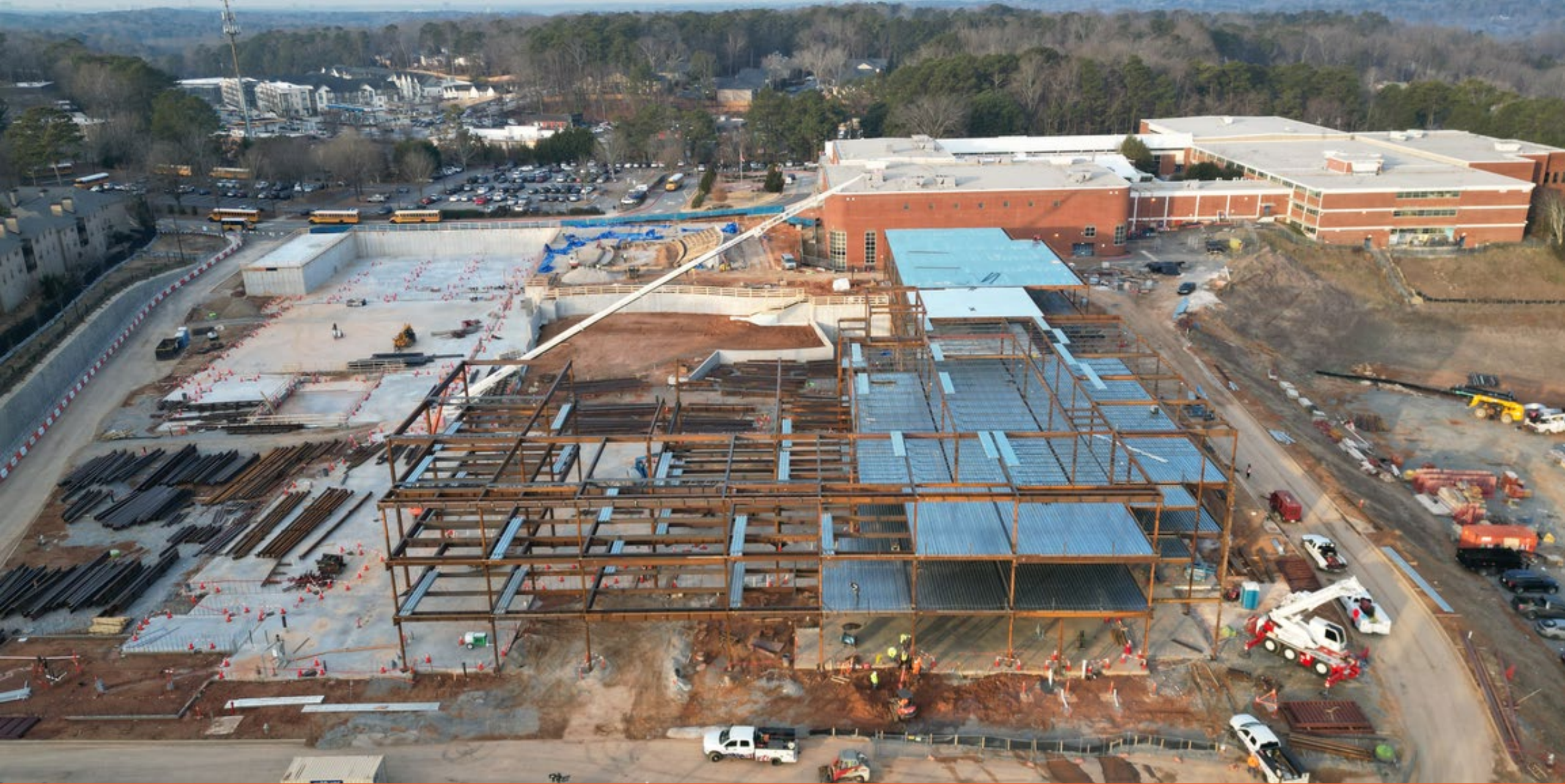
Overall Site Progress- Aerial View from South-East
