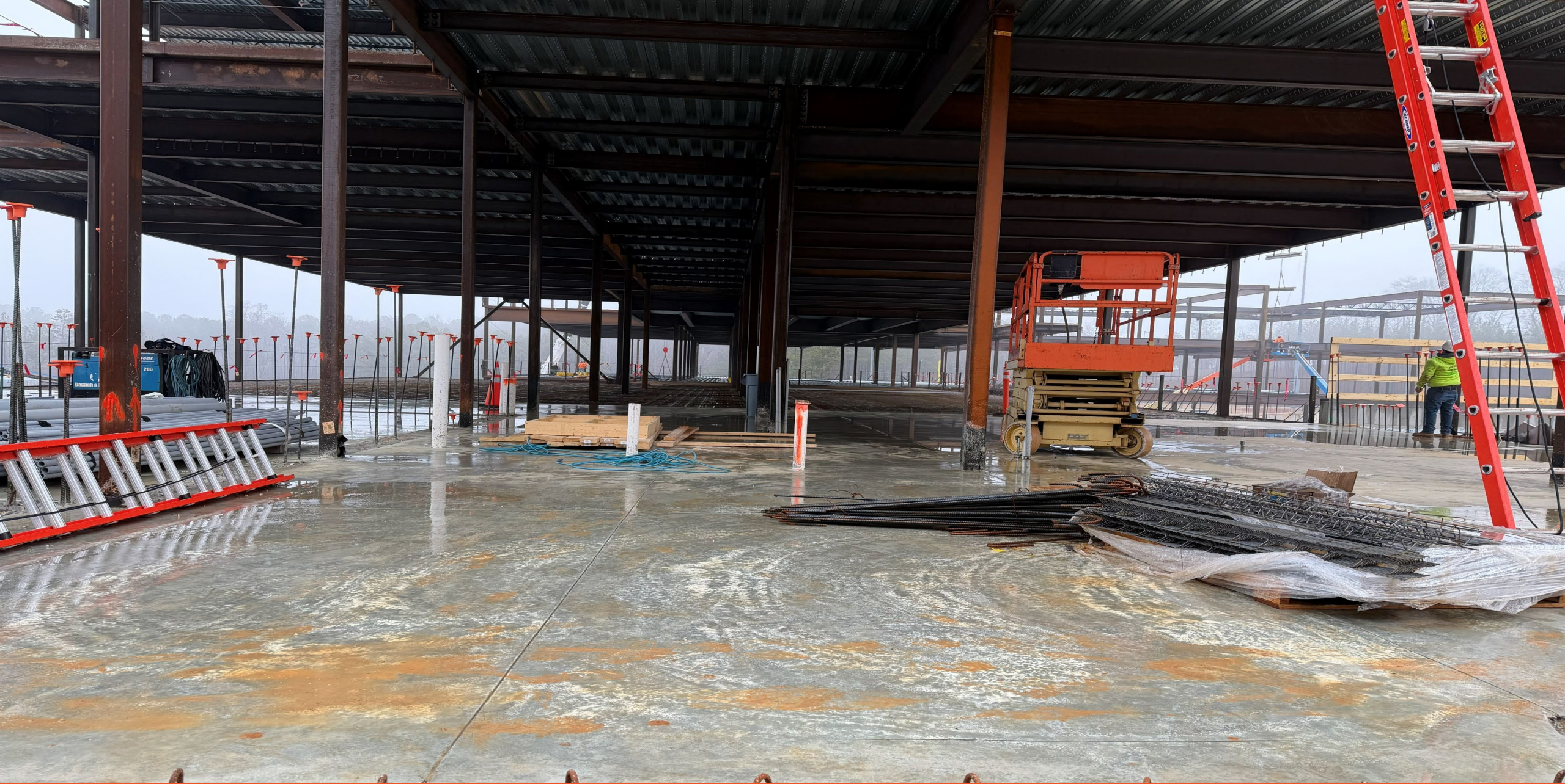
Main Building- First elevated floor slab at Area 3
