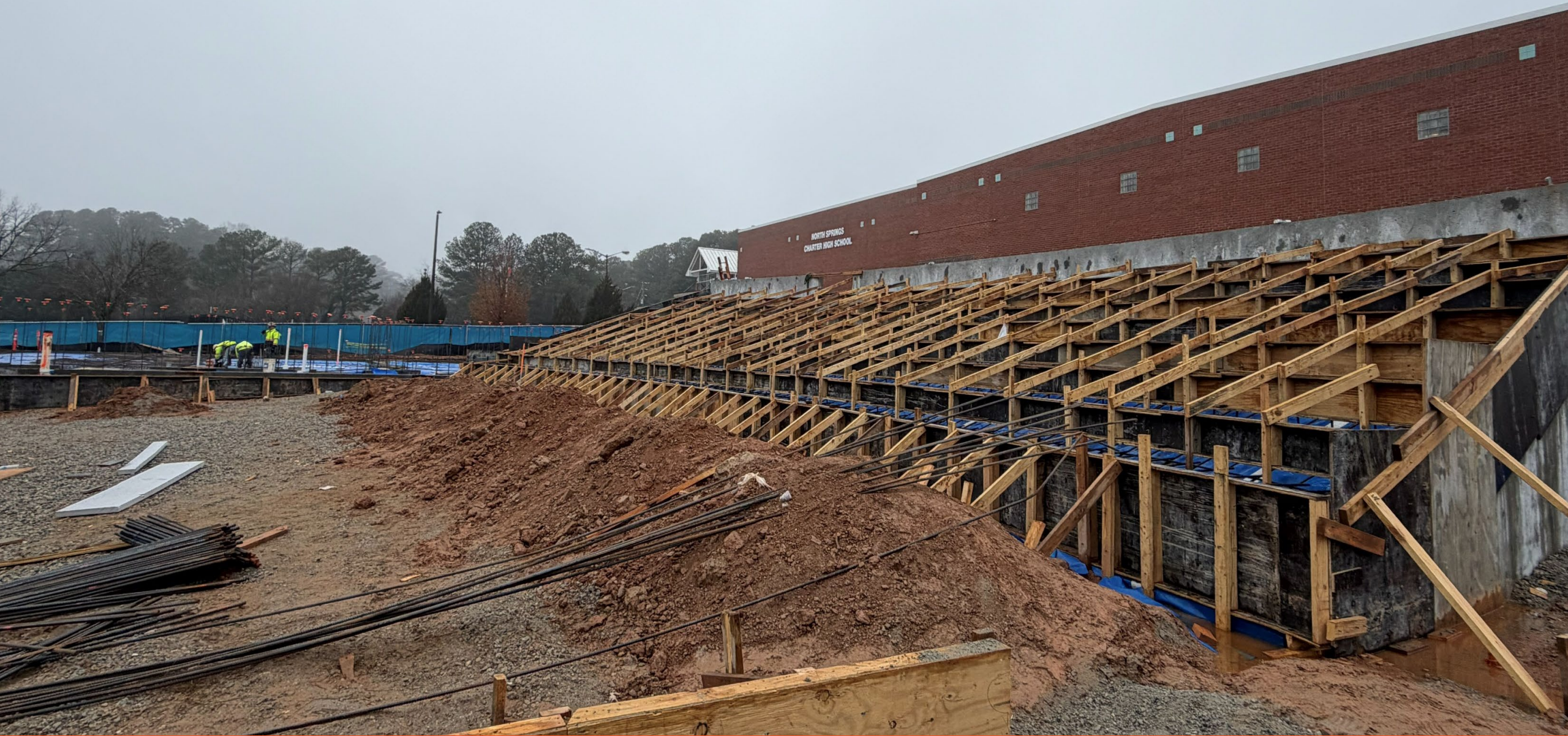
Main Building- Area 8 (Auditorium) in progress.
