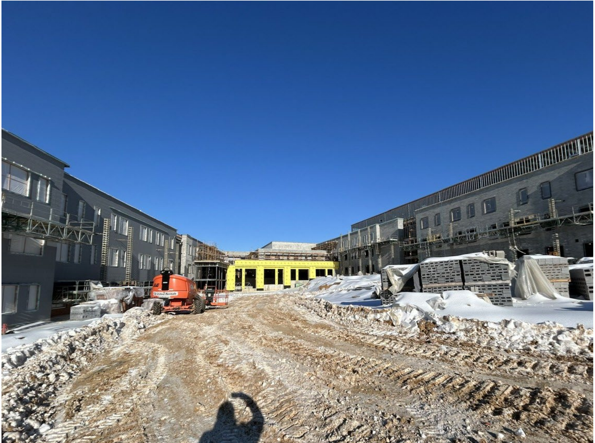
NORTH EAST MIDDLE / HIGH SCHOOL – REPLACEMENT – COURTYARD VIEW FROM BUS-LOOP
