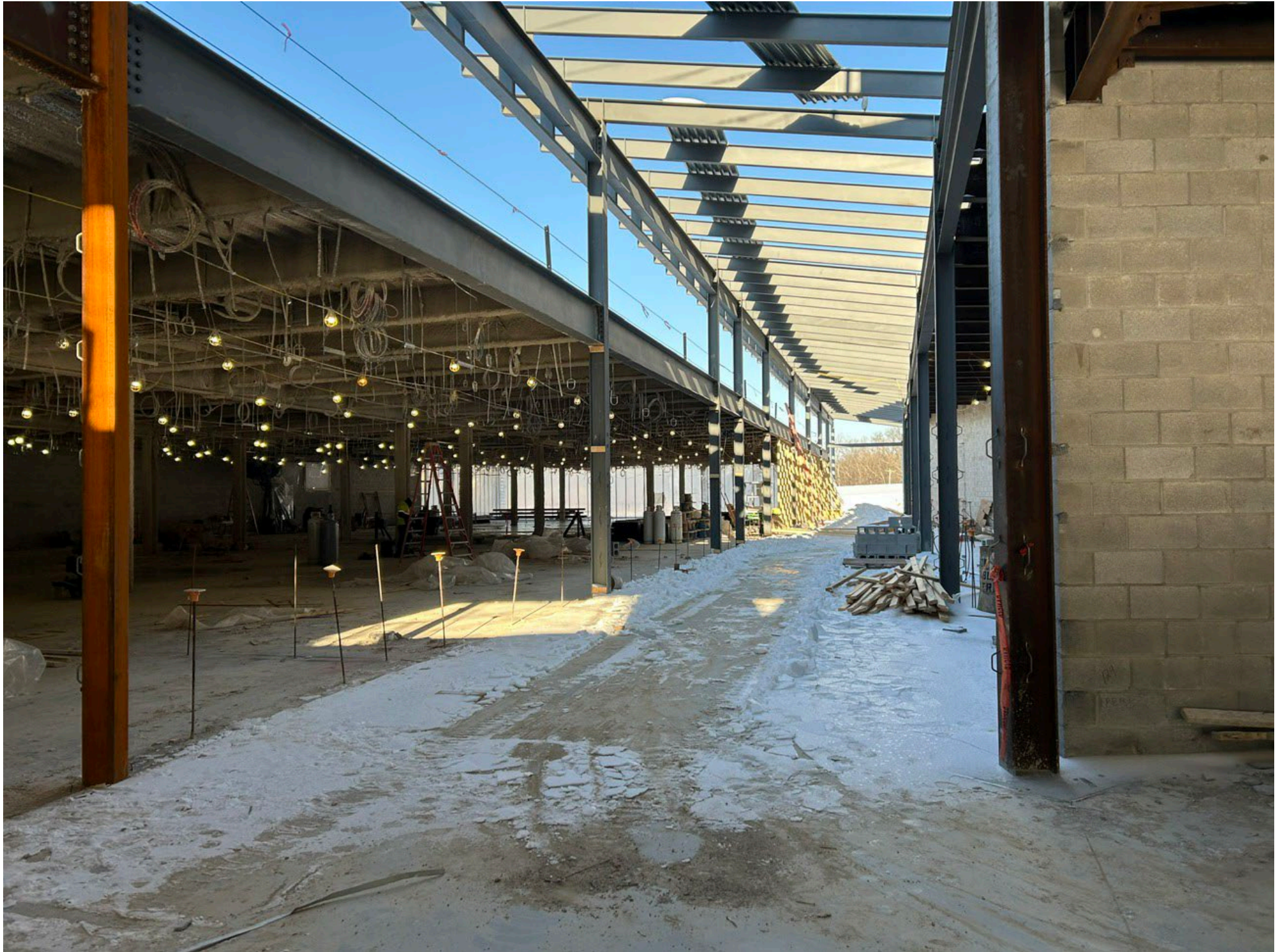
NORTH EAST MIDDLE / HIGH SCHOOL – REPLACEMENT – MAIN “BOARDWALK” CORRIDOR / ADMIN AREA
