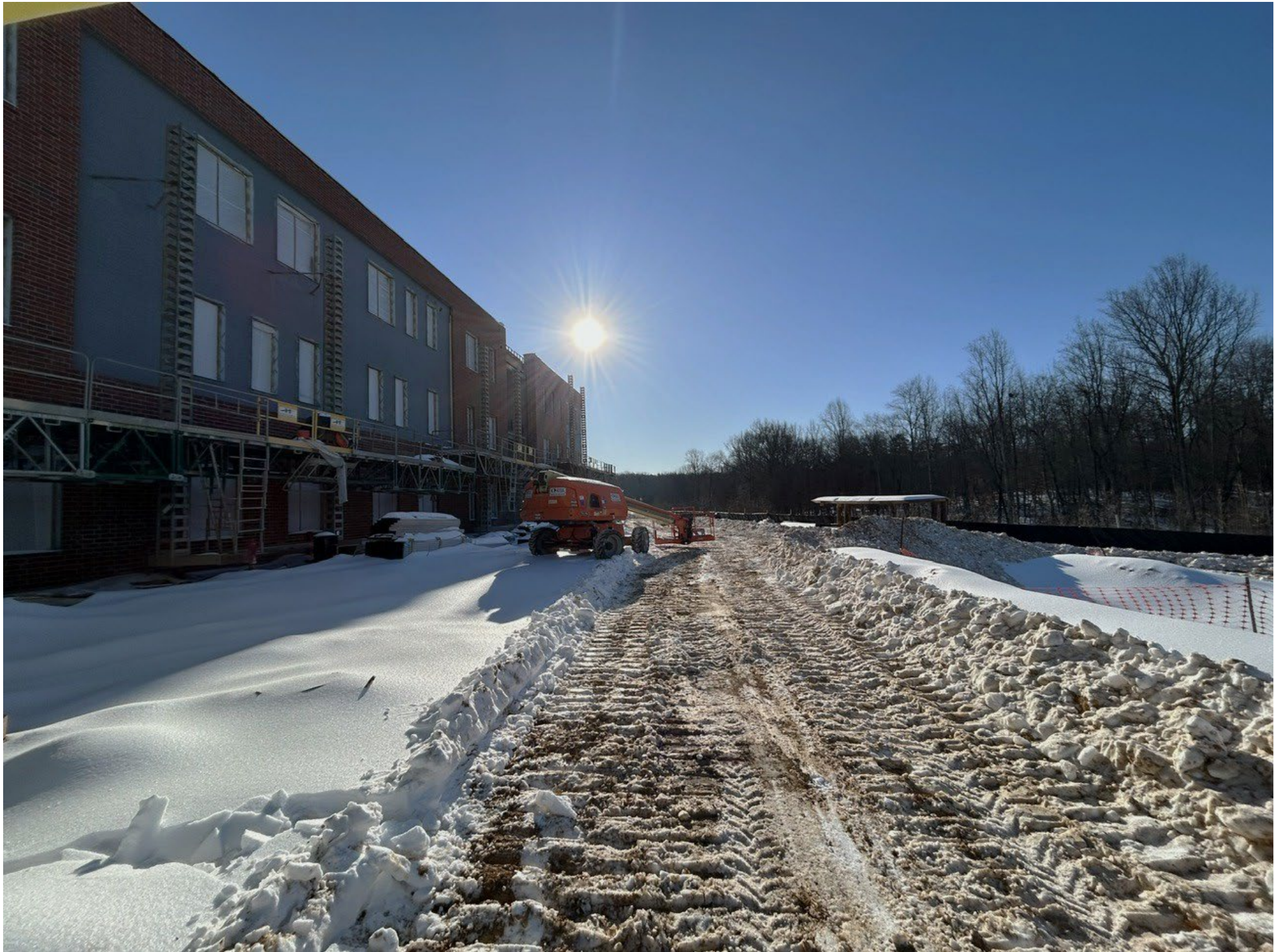
NORTH EAST MIDDLE / HIGH SCHOOL – REPLACEMENT – BRICK VENEER INSTALLATION – AREA C – MIDDLE SCHOOL WING
