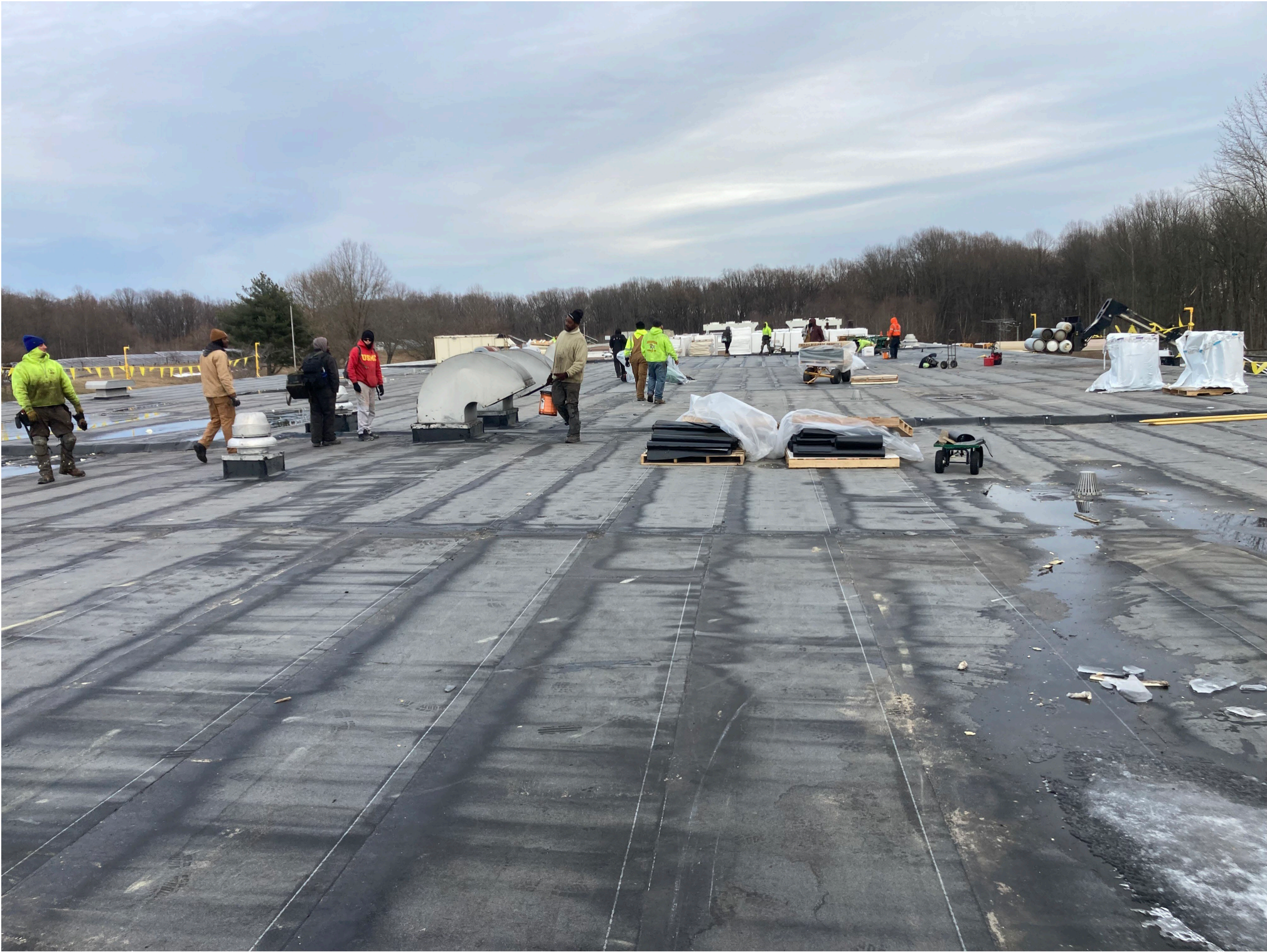
ADMINISTRATIVE SERVICES CENTER – ROOF REPLACEMENT
