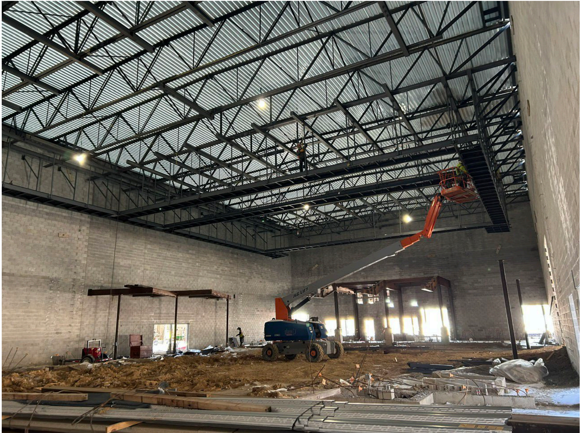
NORTH EAST MIDDLE / HIGH SCHOOL – REPLACEMENT – AUDITORIUM CATWALK
