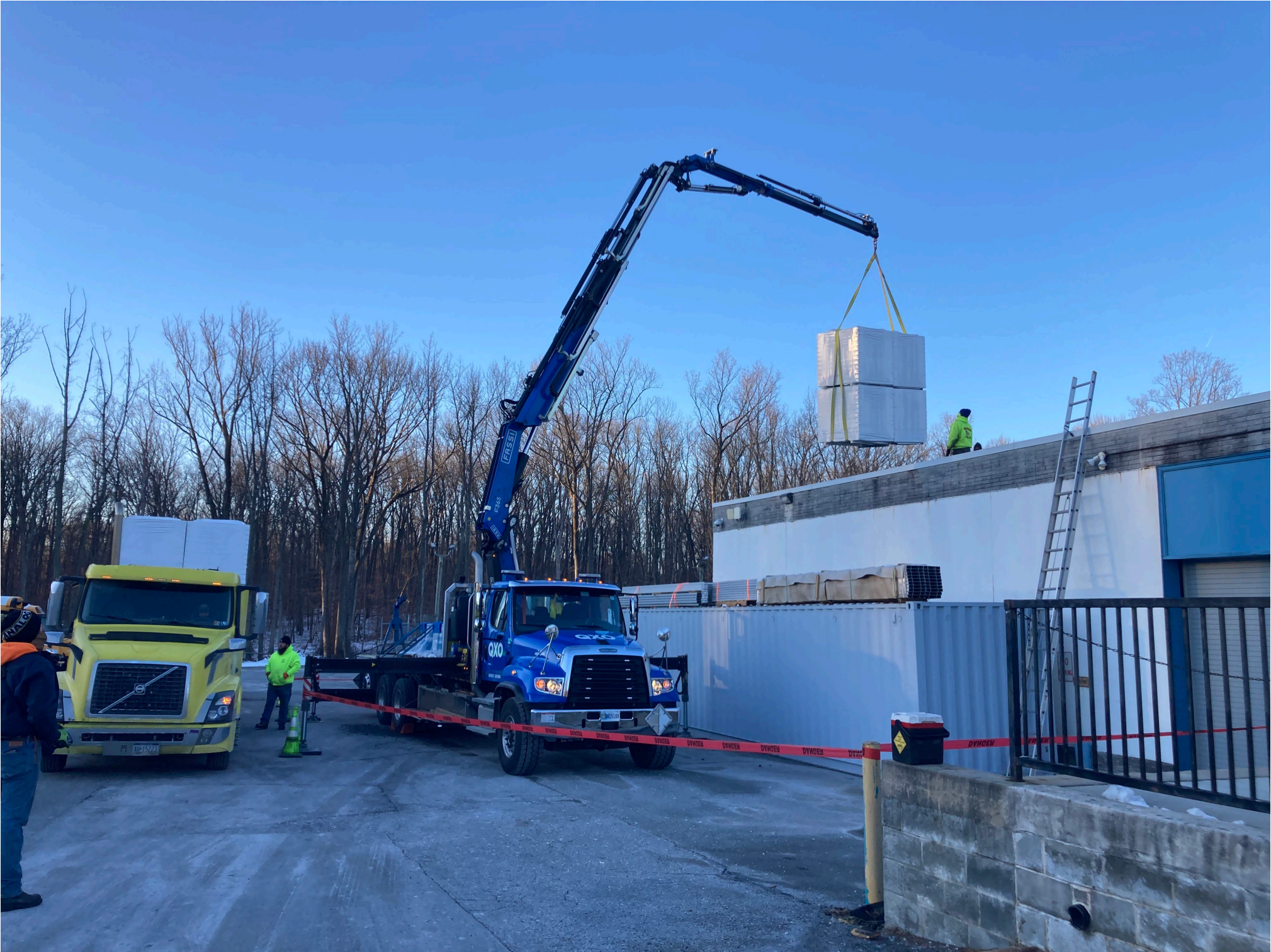
ADMINISTRATIVE SERVICES CENTER – ROOF REPLACEMENT
