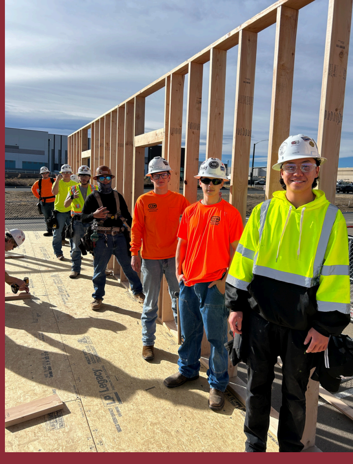
Year 2 - First Wall Lift
