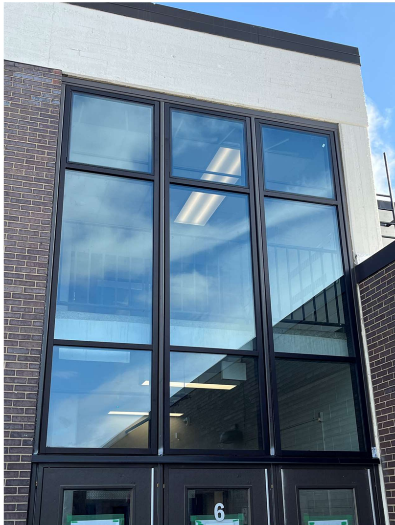
Clague Middle School Window Replacement
