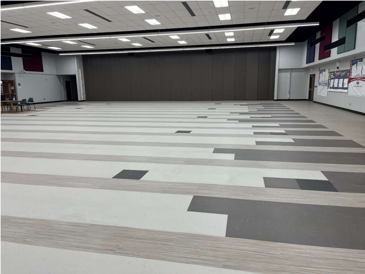
Scarlett Middle School Cafeteria Floor Replacement
