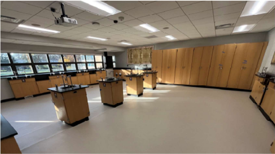
Classroom Flooring Replacement
