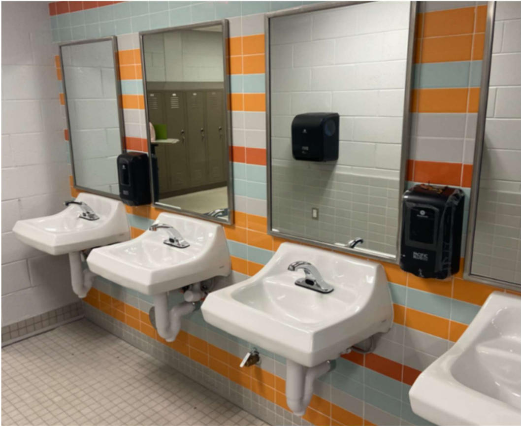
Scarlett Middle School Restroom Improvements
