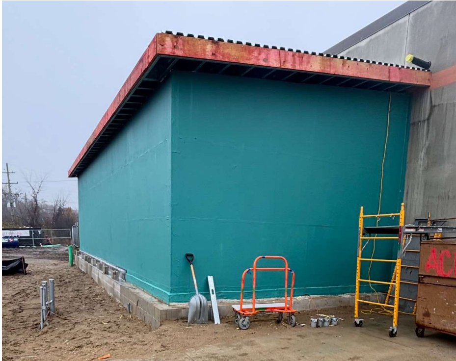
Network Operations Center (NOC)
