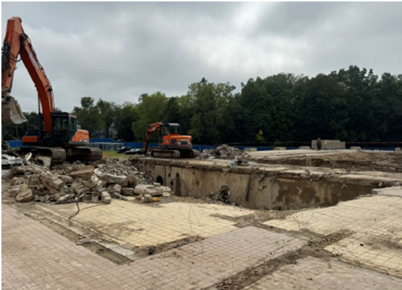
Slauson Middle School Pool Demolition
