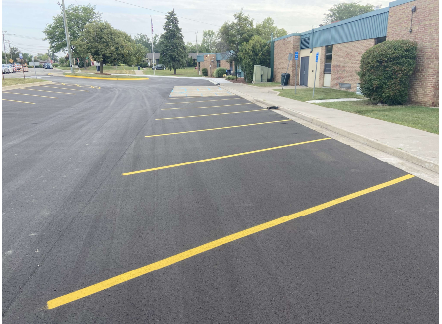
Pittsfield Elementary Paving Improvements
