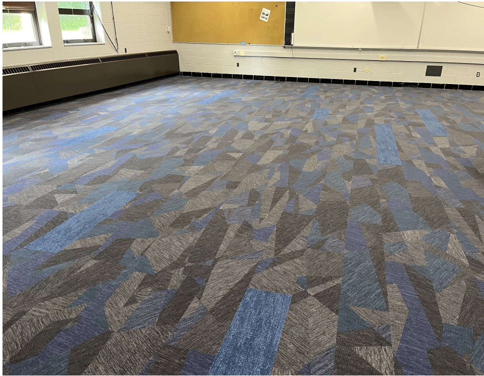
Scarlett Middle School Floor Replacement
