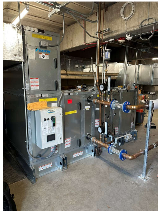
Haisley Elementary – HVAC Improvements
