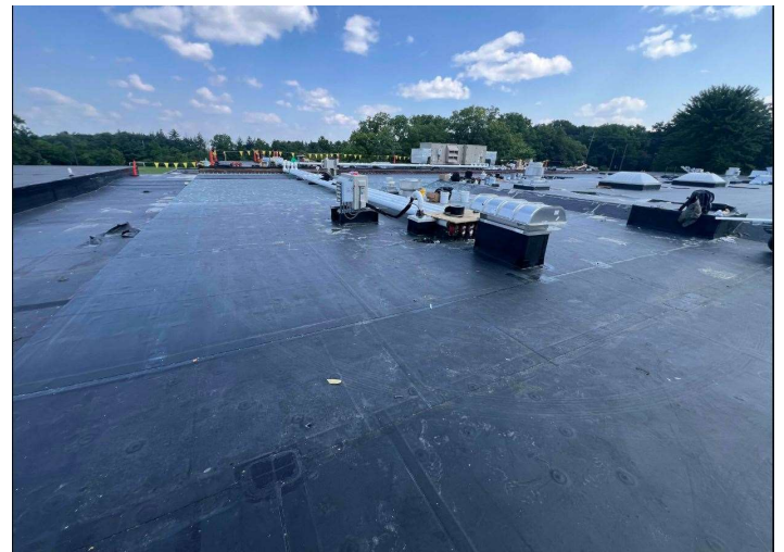
Forsythe Middle School Roofing
