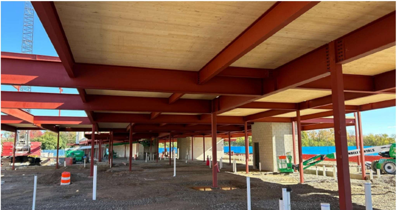
Cross Laminated Timber – CLT 2 nd Floor
