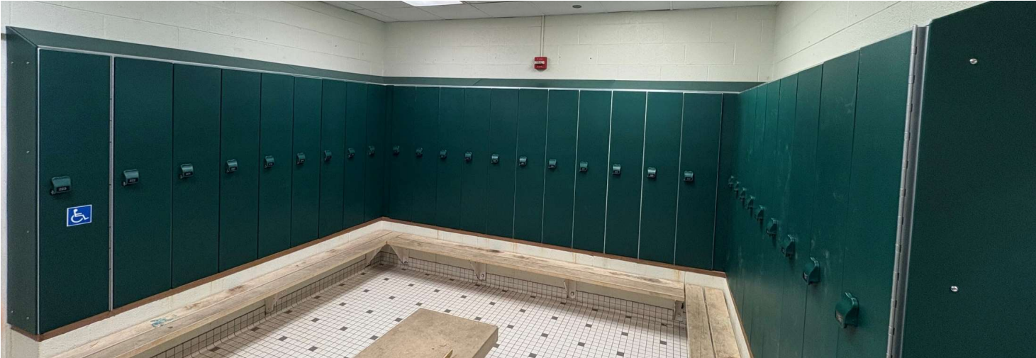
Huron High School Pool Locker Replacement
