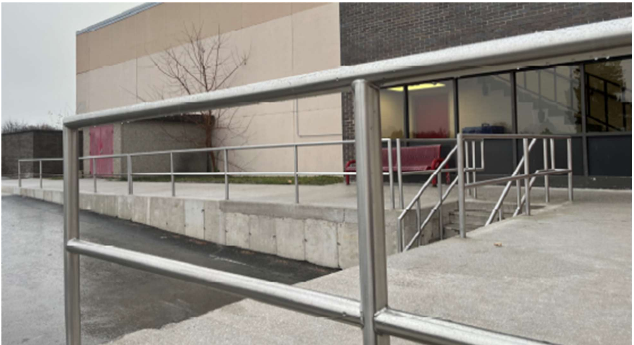
Scarlett Middle Loading Dock Improvements
