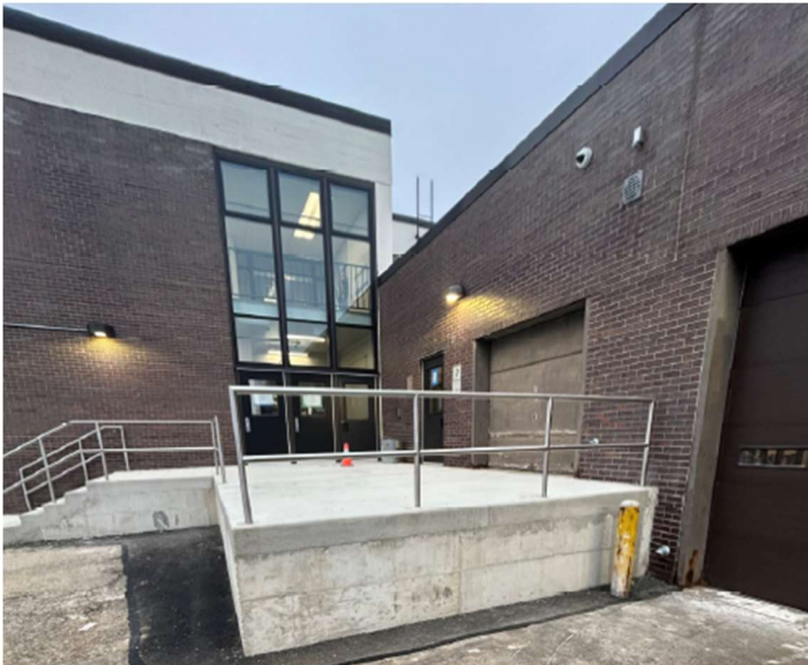
Scarlett Middle Loading Dock Improvements
