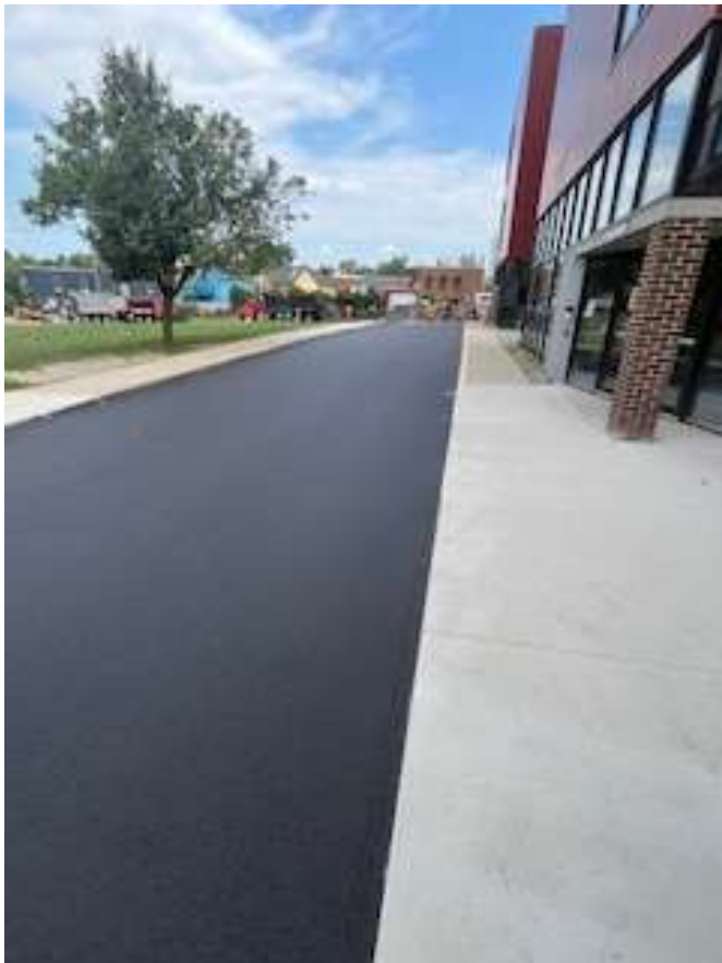
Community High School Paving Improvements
