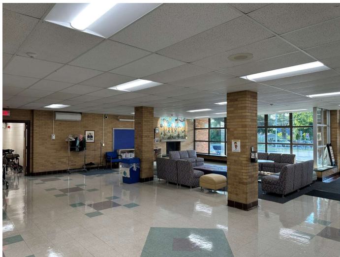
Haisley Elementary Air Conditioning & Lighting
