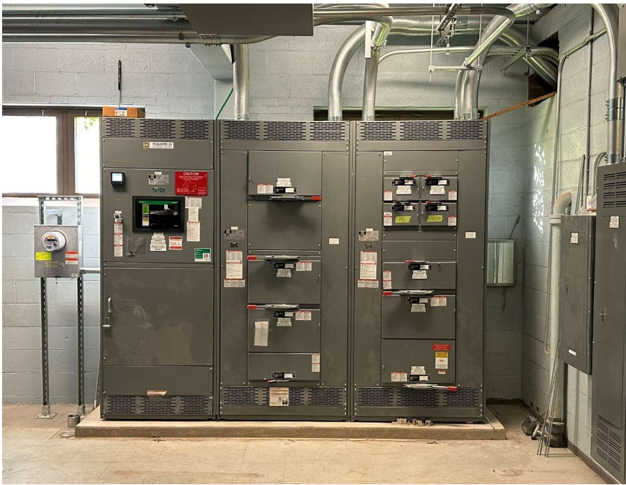
Haisley Elementary – Electrical Upgrade
