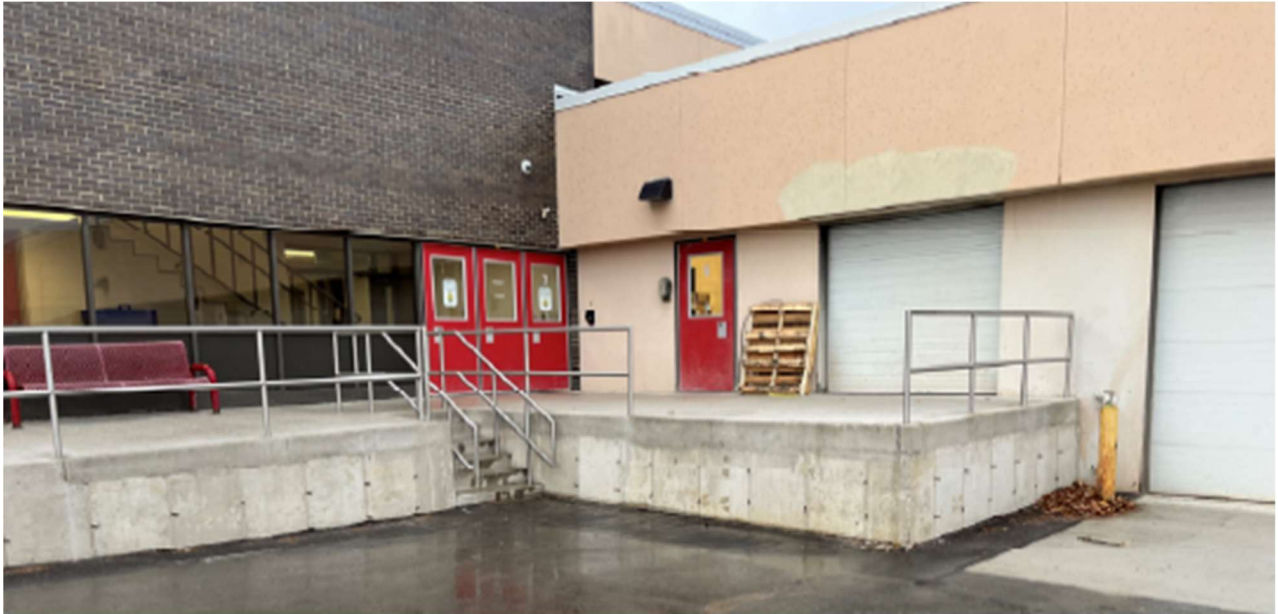
Scarlett Middle Loading Dock Improvements
