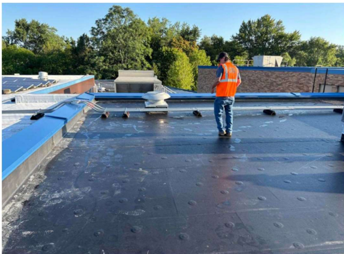
Ann Arbor Steam Roofing
