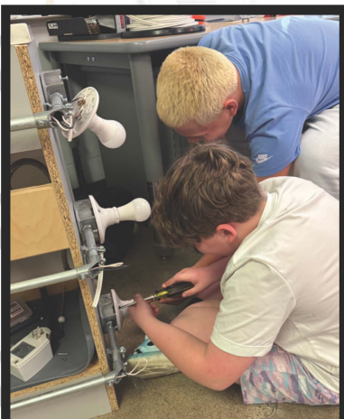
Students learn fundamental electrical wiring skills by splitting and connecting wires to power a light bulb.
