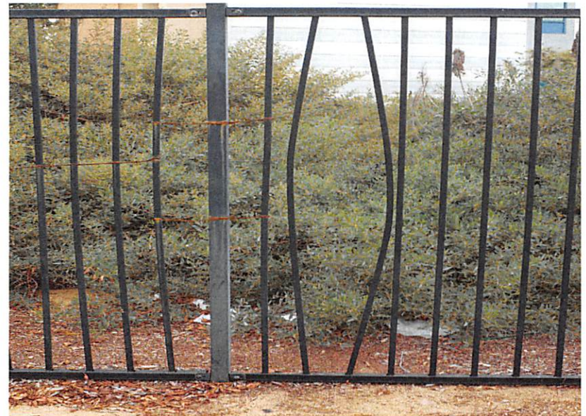
Fencing at Willow Elementary School
