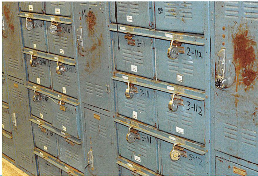
Boys' Locker Room at San Ysidro Middle School
