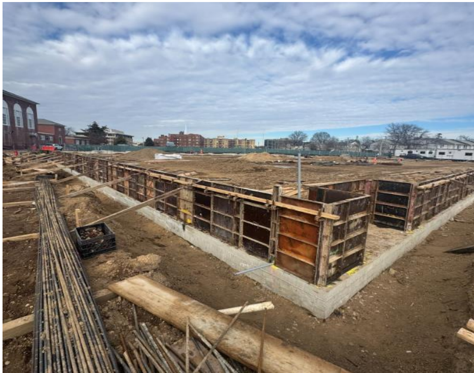
Hempstead ABGS MS – Foundation wall Forms/Rebar
