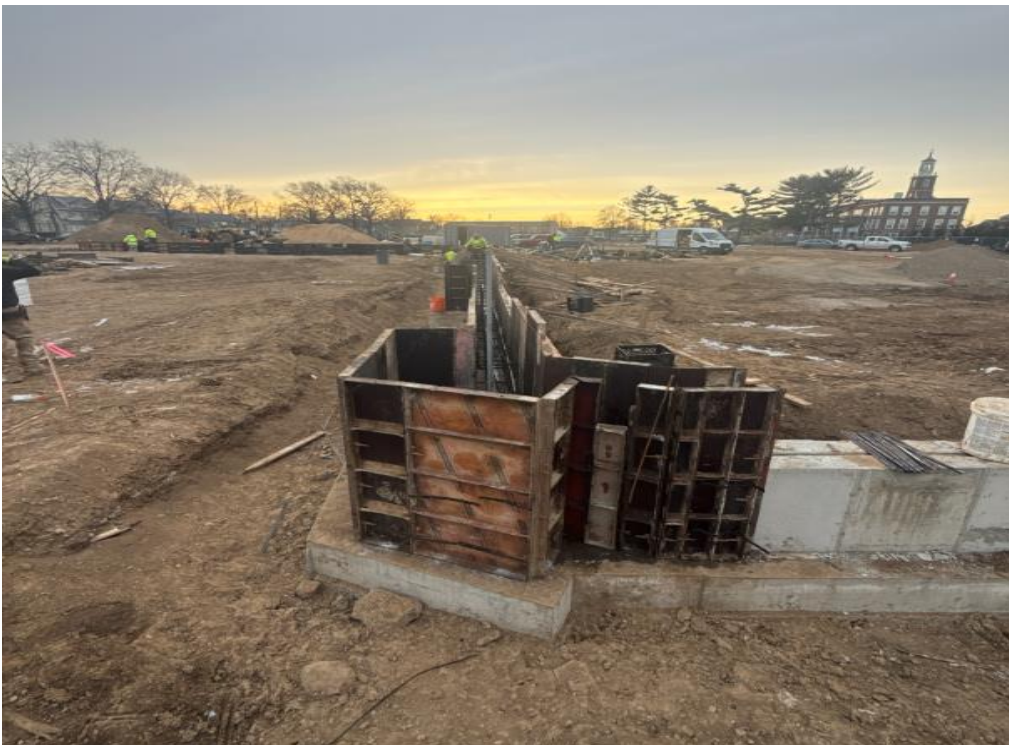
Hempstead ABGS MS – Foundation wall Forms/Rebar
