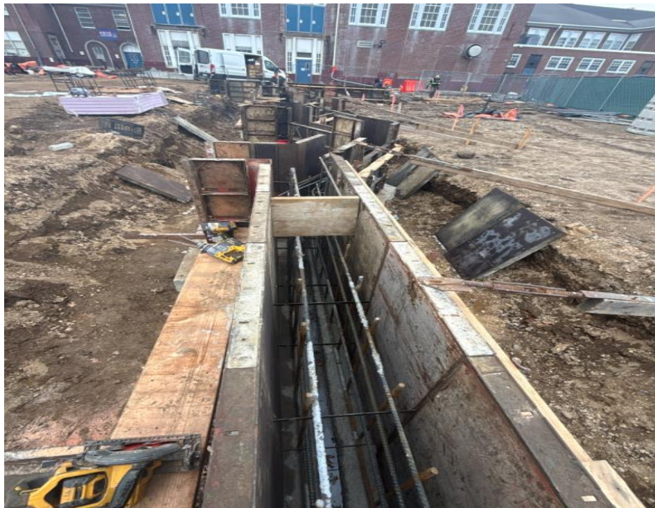
Hempstead ABGS MS – Foundation wall Forms/Rebar
