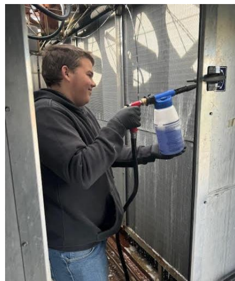
Dylan Holmes in HVAC working at Pierce Refrigeration
