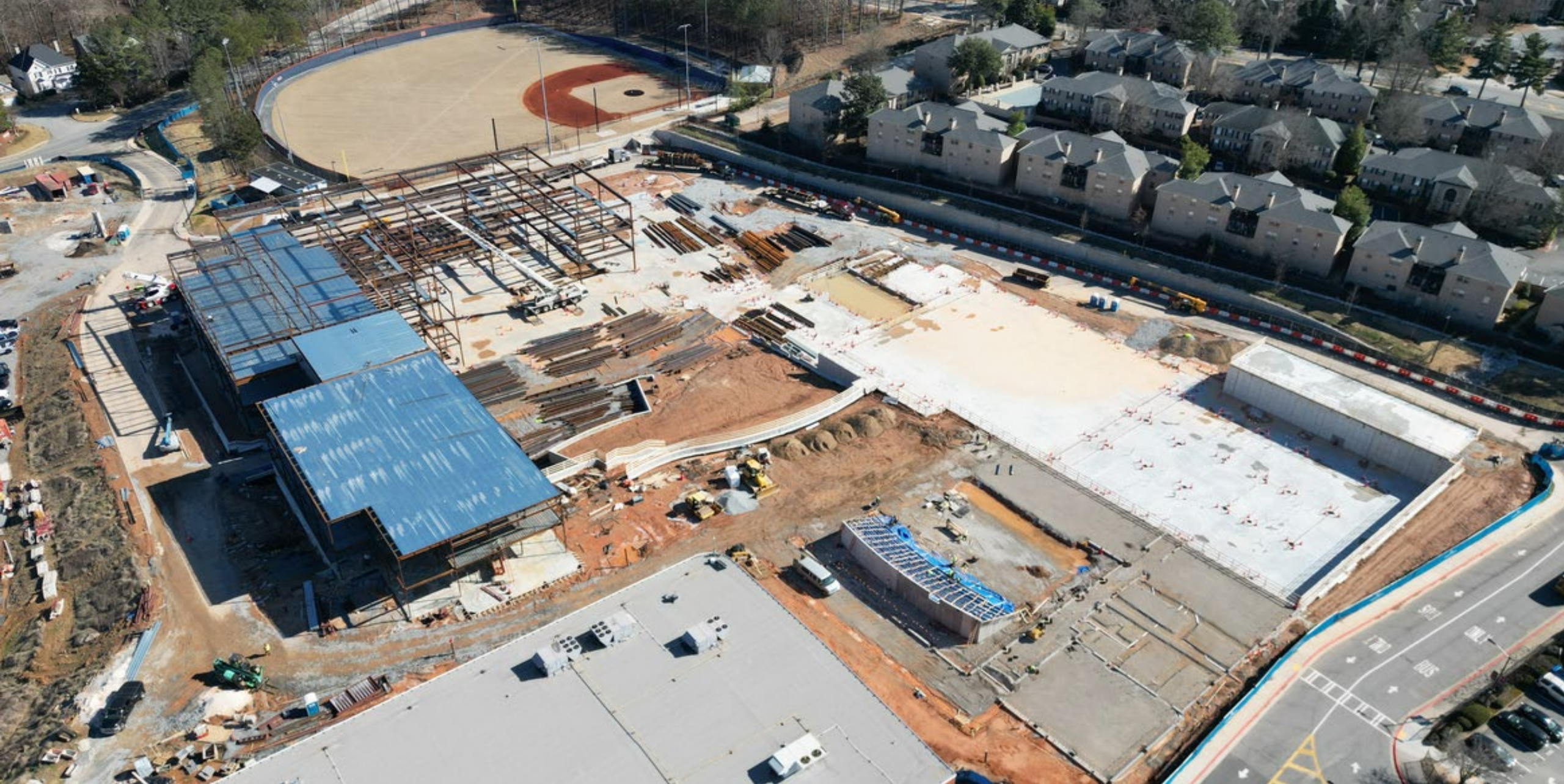
Overall Site Progress - Aerial view from North-West
