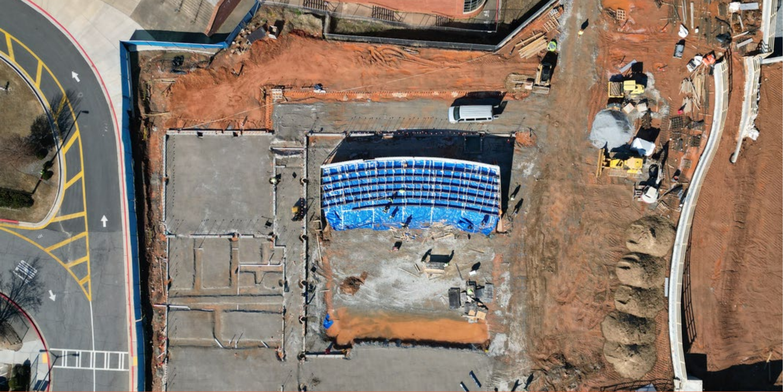
Main Building - Area 8 (Auditorium) in progress
