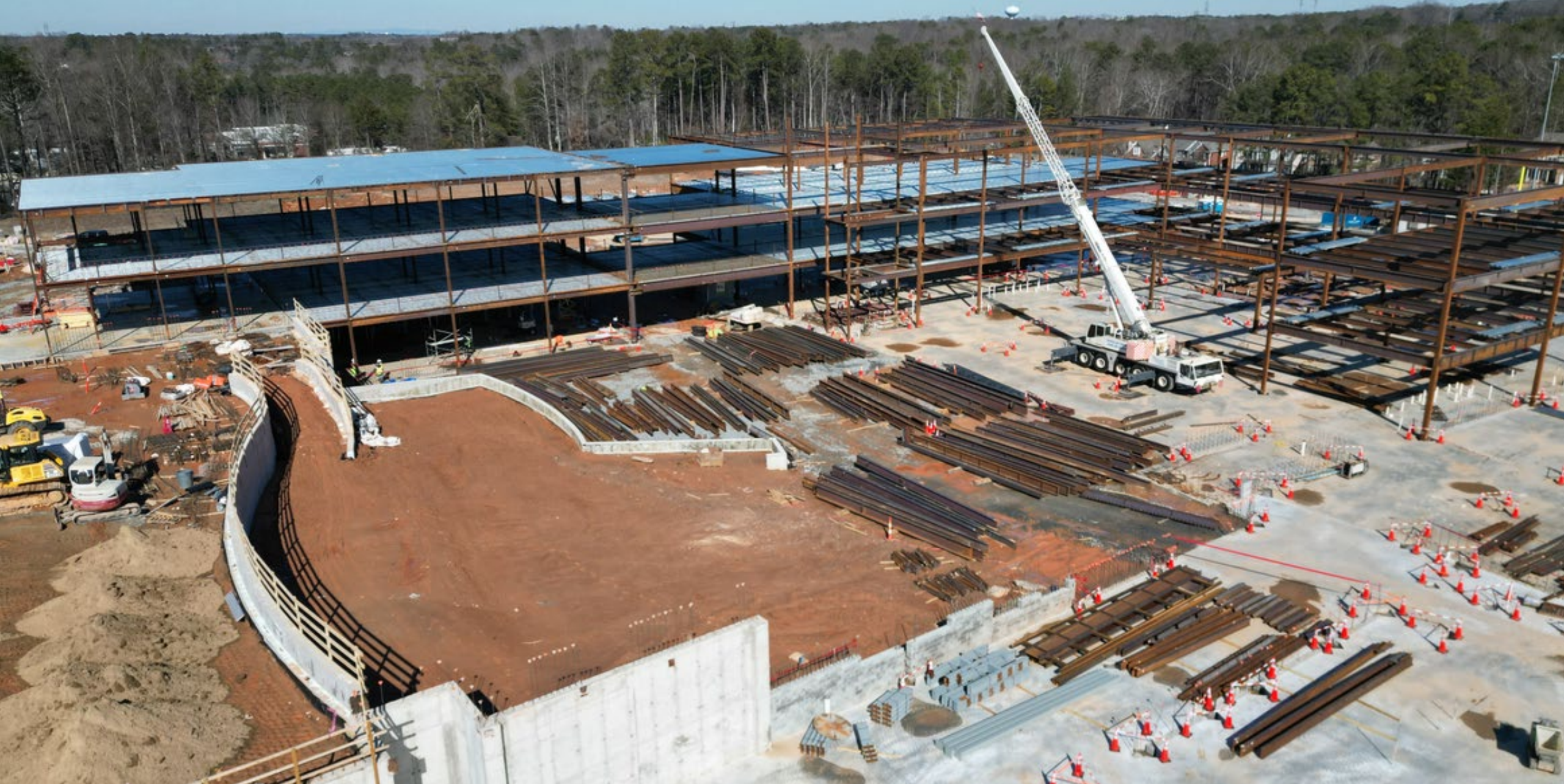
Main Building - Courtyard Retaining Walls and Steel Erection
