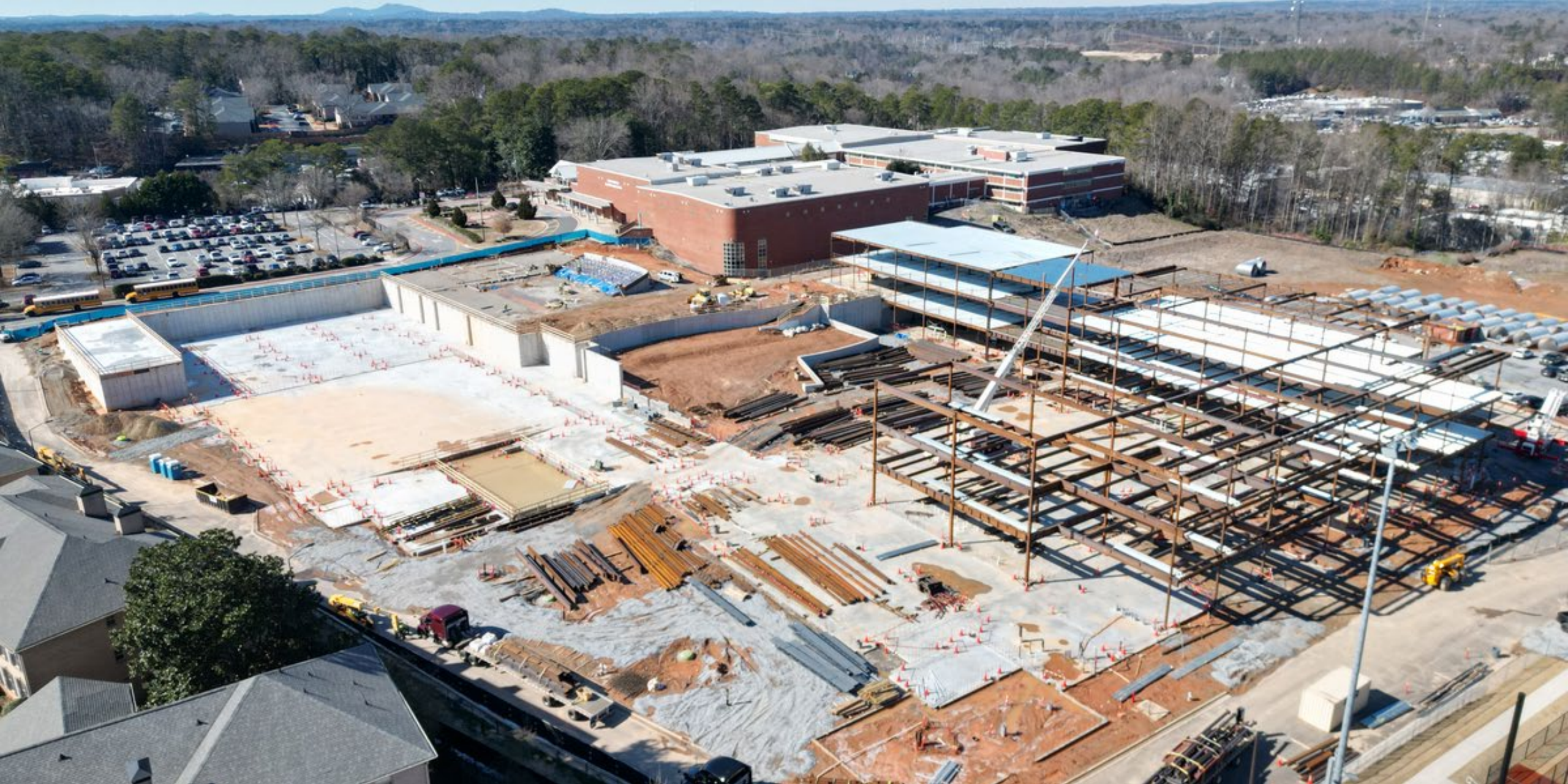
Overall Site Progress - Aerial View from South-East
