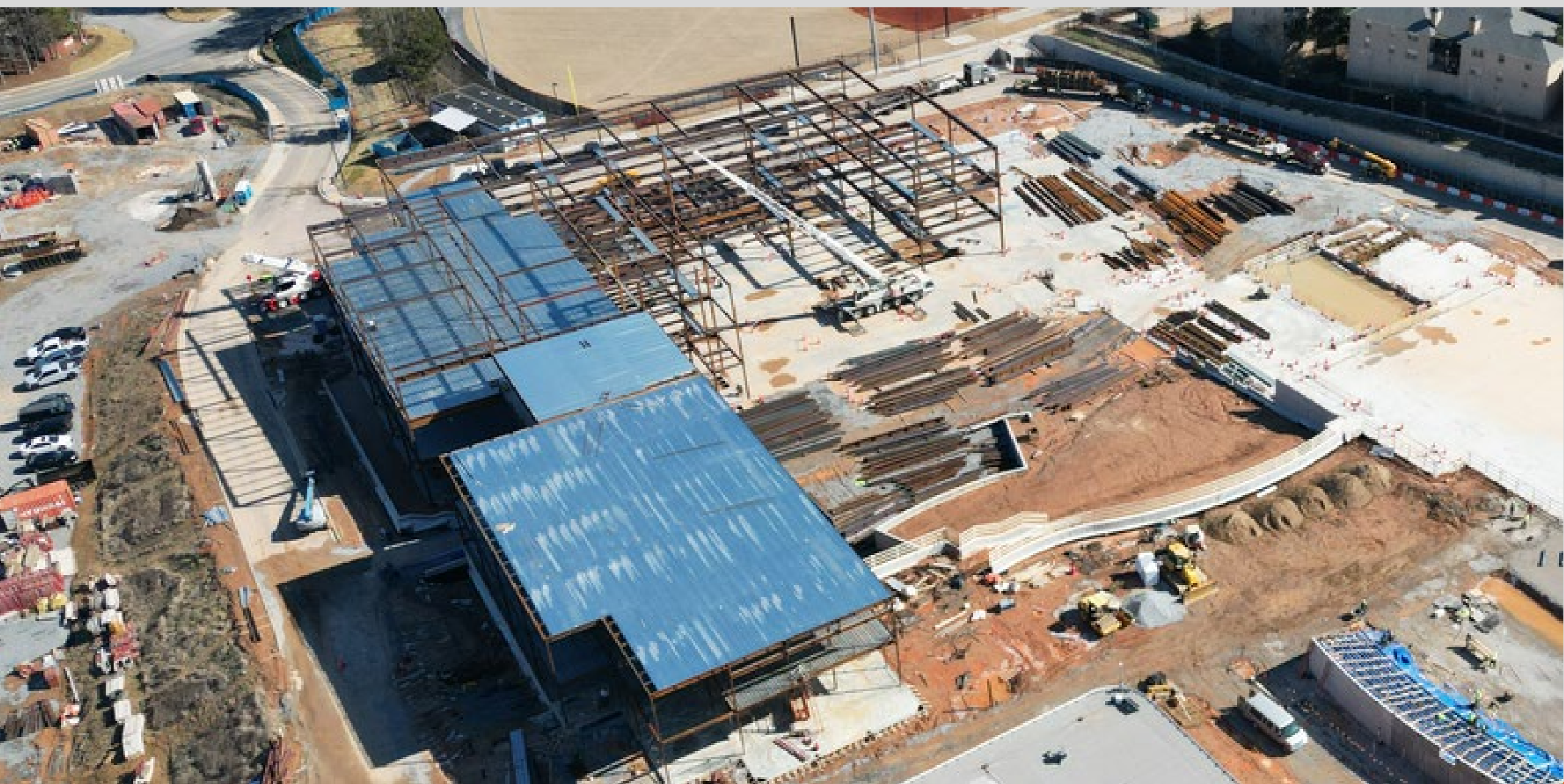
Roof Decking started on site
