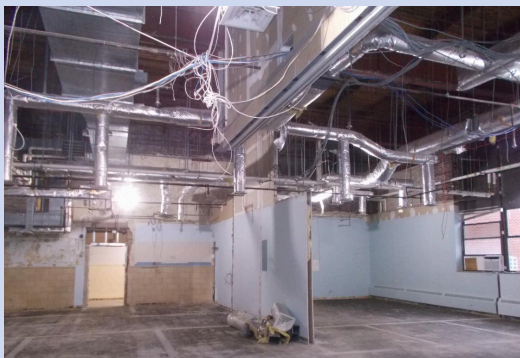
Selective demolition has been completed in the first floor of the La Grande building.
