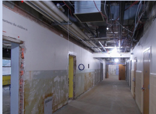
Selective demolition has been completed in the first floor of the La Grande building.
